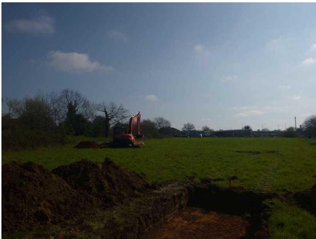
Photograph 1 Site shot view north-east.
