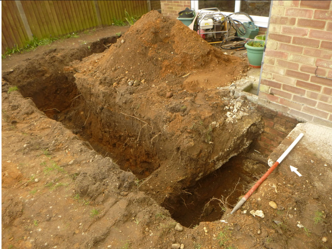
Photograph 1 General foundation trench shot, looking north.
