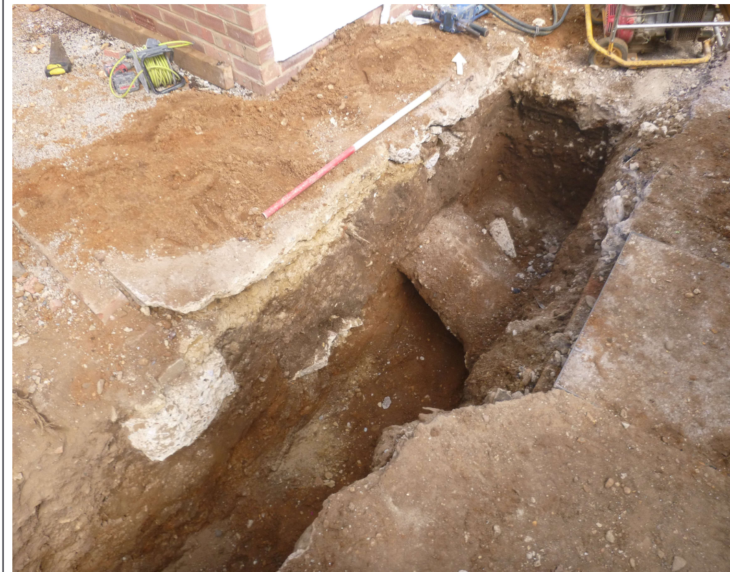
Photograph 4 Concrete and services in section with scale, looking north.
