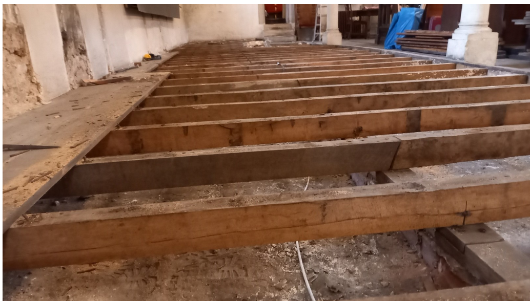
Photograph 1 General shot of wooden battens and bricks after floorboards removed in north aisle. Taken by Bakers of Danbury.
