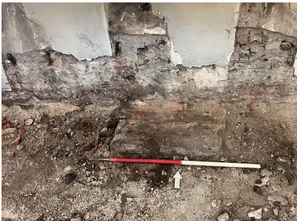
Photograph 5 View of F4, looking north.
