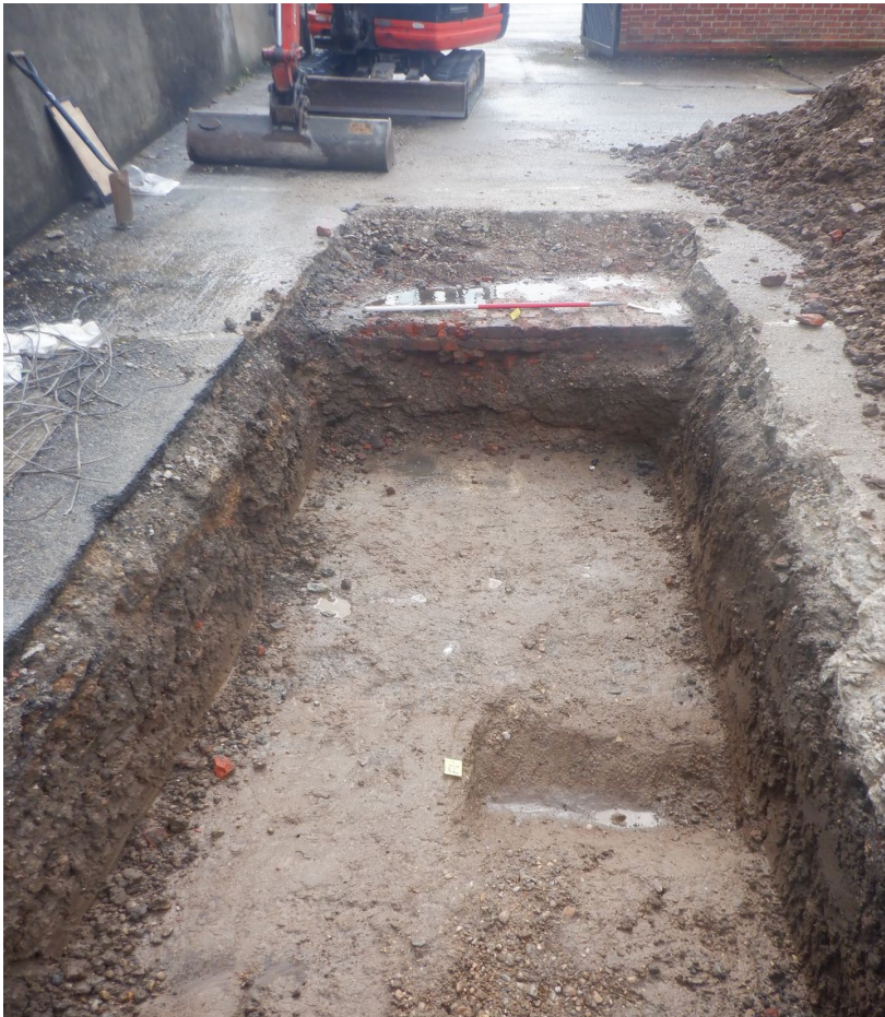
Photograph 1 Trench 1, F3 facing south-east.
