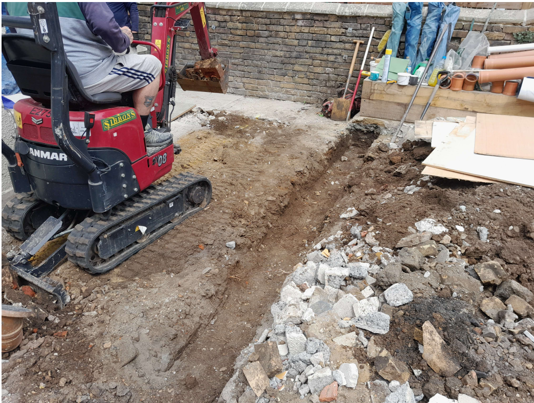
Photograph 4 General shot of retaining wall foundation, looking north.
