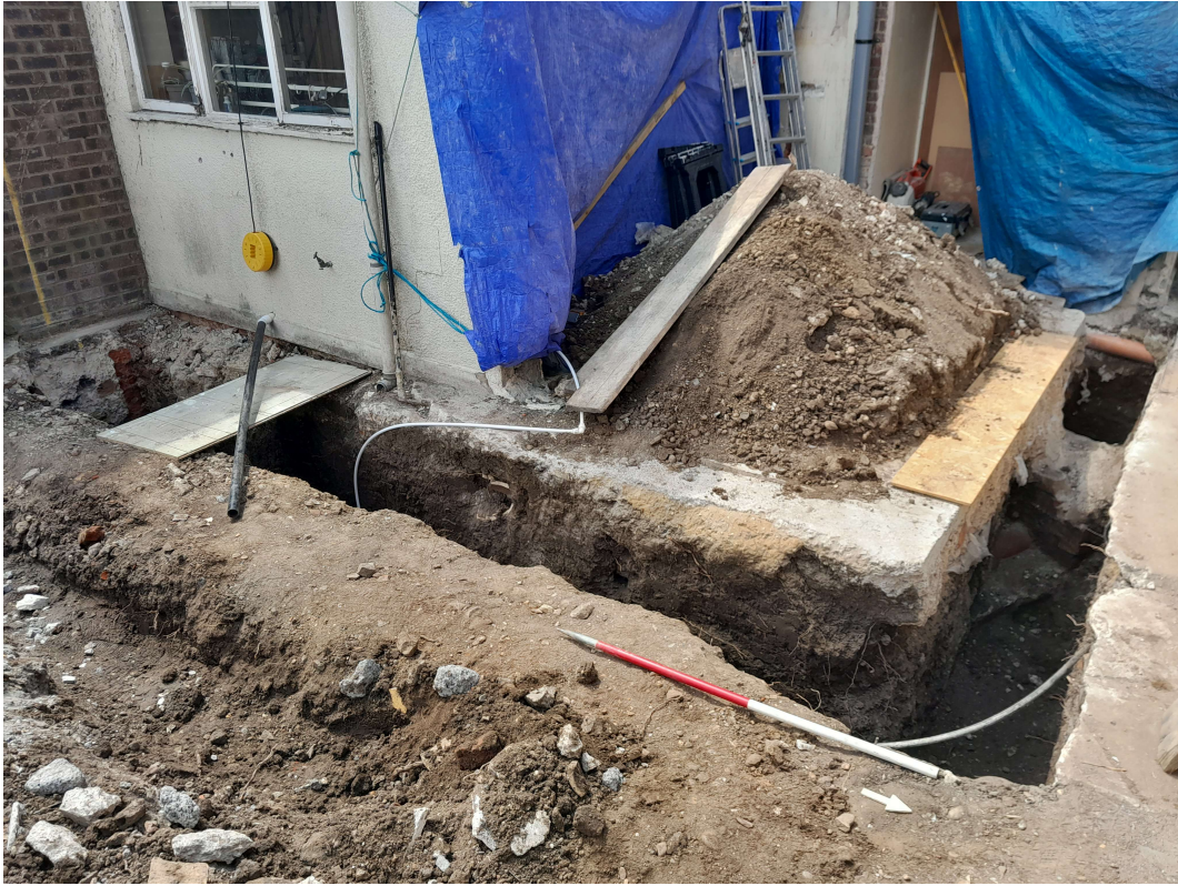
Photograph 1 General view of foundation trench, looking south-west.
