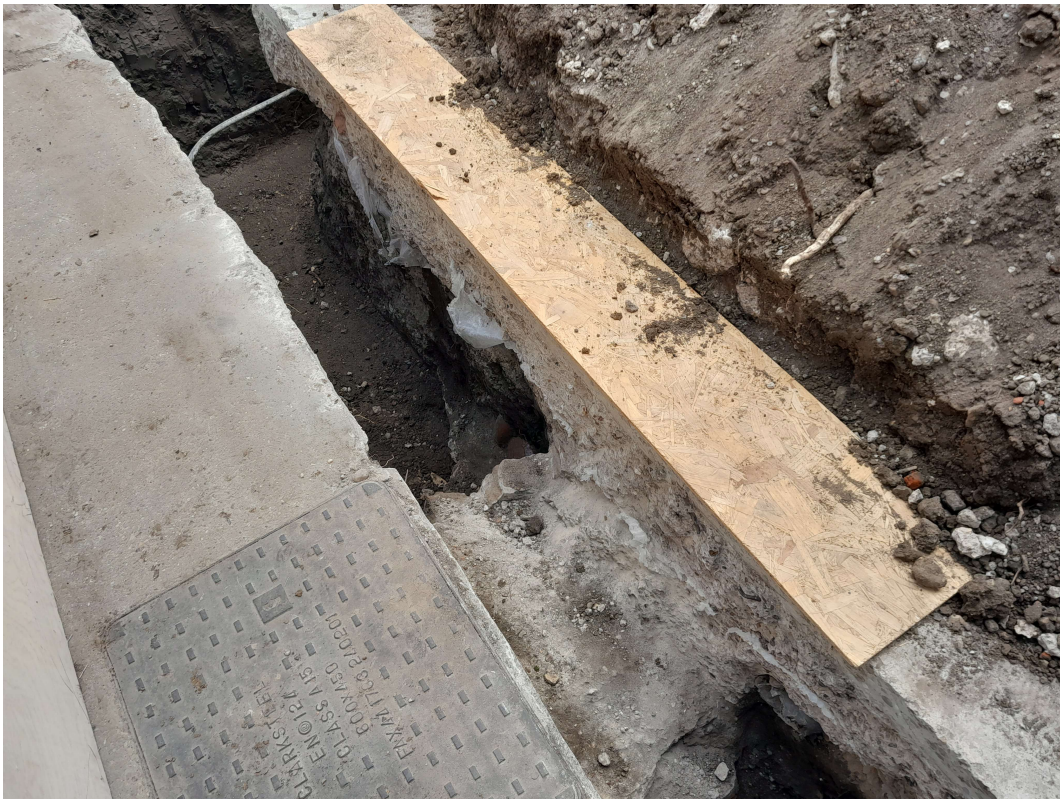
Photograph 2 Modern service in foundation trench, looking south-east.
