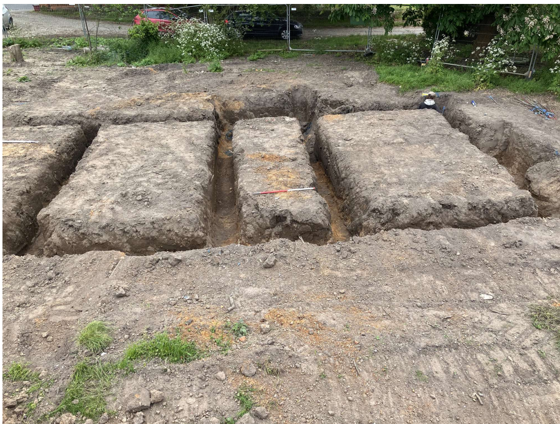
Photograph 6 Foundation trenches, looking east-south-east.
