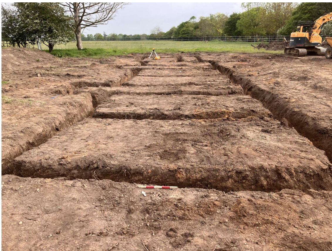
Photograph 1 Foundation trenches, looking north.
