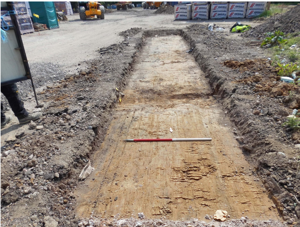
Photograph 5 Trench 3, looking south.
