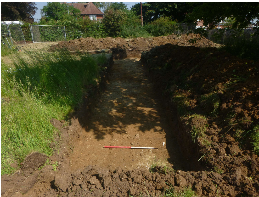
Photograph 2 Trench 2, looking north.
