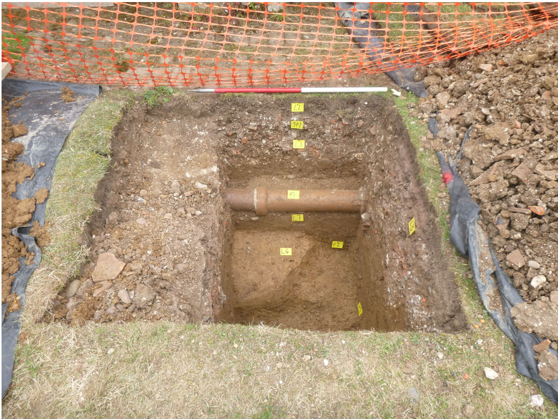
Photograph 6 Test-pit 2, looking south-west.
