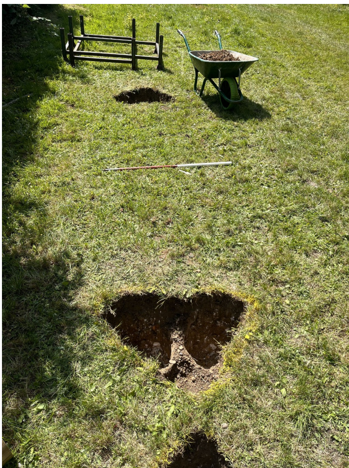
Photograph 12 Overall view of post-holes for shimmy ropes, view south-west.
