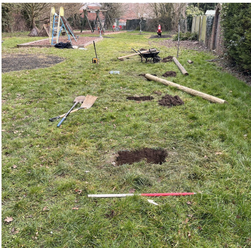
Photograph 2 Post-holes for obstacle course from south end, view north-east.
