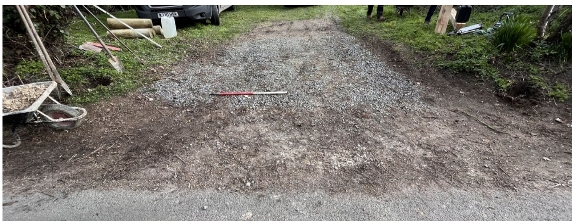
Photograph 4 Overall shot of entrance gate-posts, view north-east.
