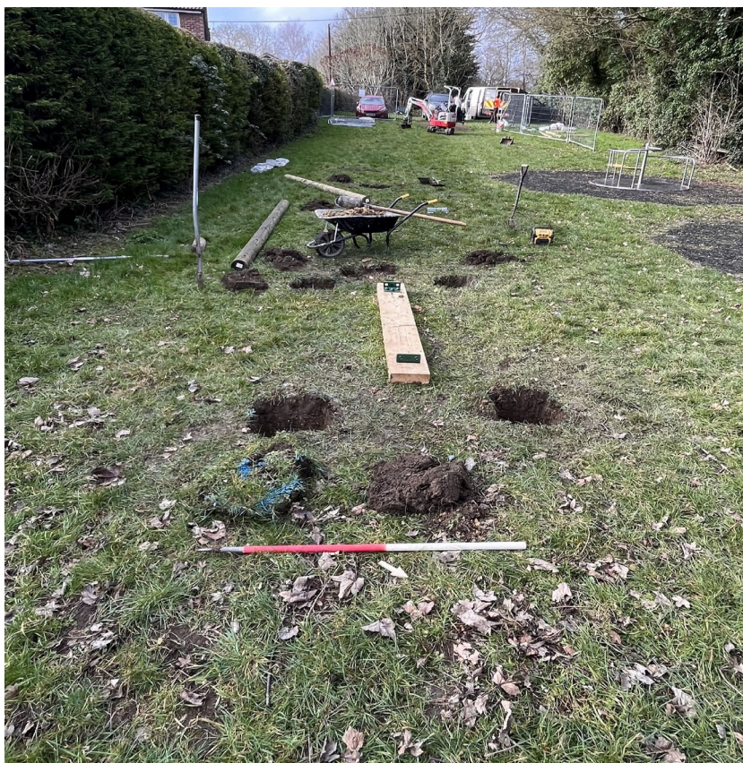
Photograph 1 Post-holes for obstacle course from north end, view south-west.
