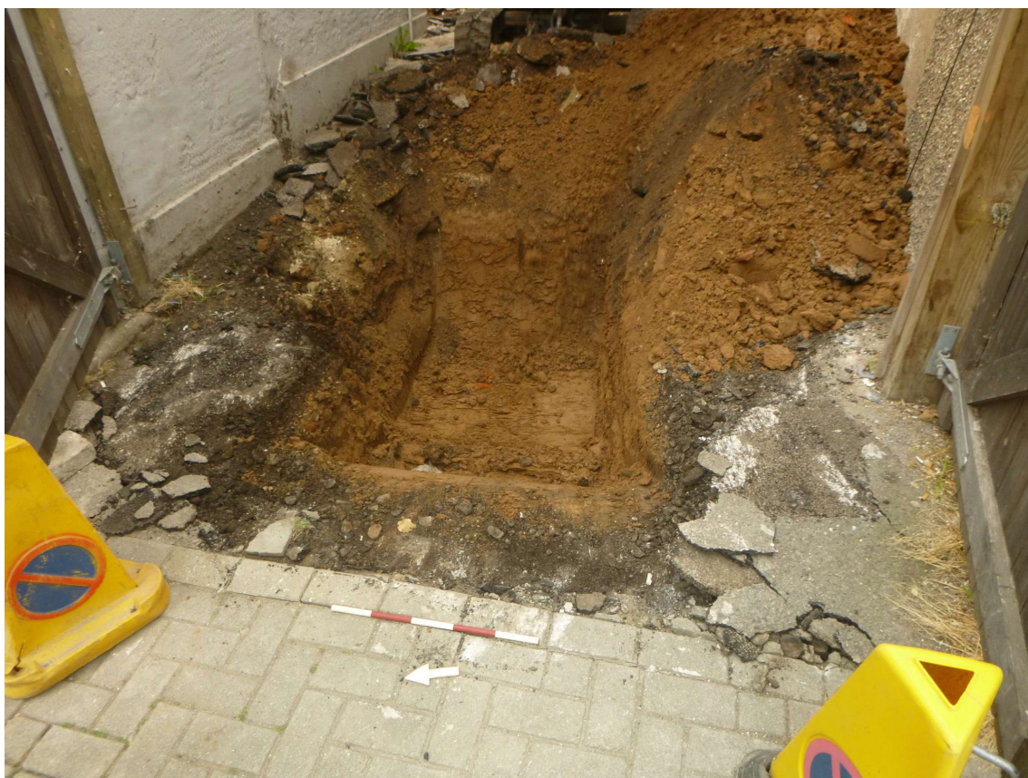
Photograph 6 Test-pit at front of property, looking south-east.
