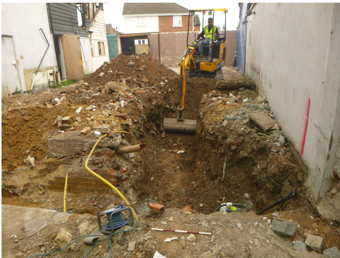
Photograph 5 Working shot, looking south-east.
