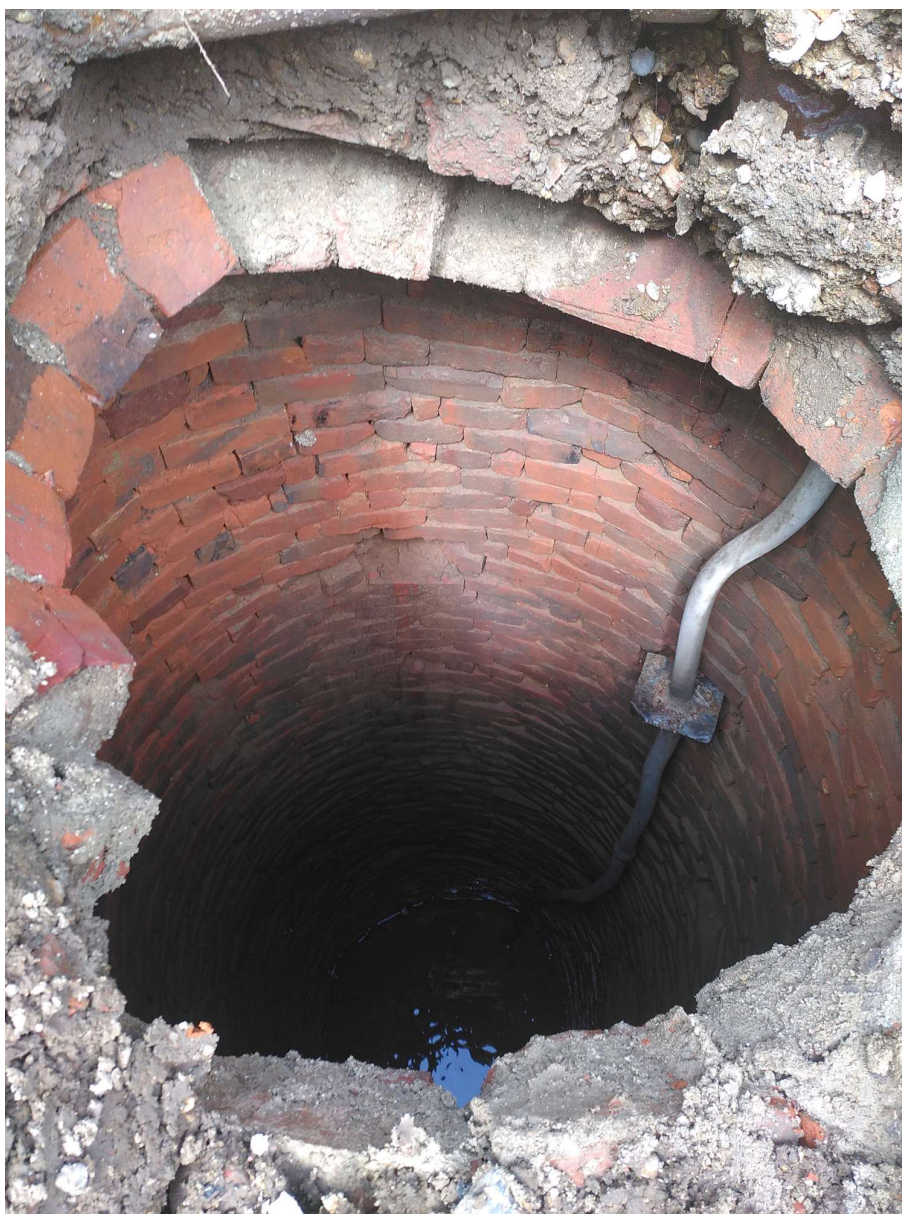
Photograph 7 Brick-lined well F6 with lead pump, looking north.
