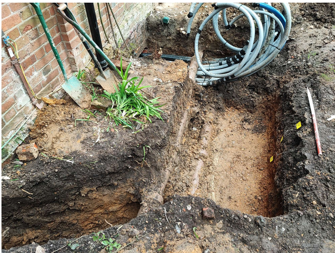
Photograph 2 Trench adjoining house, looking north-west.
