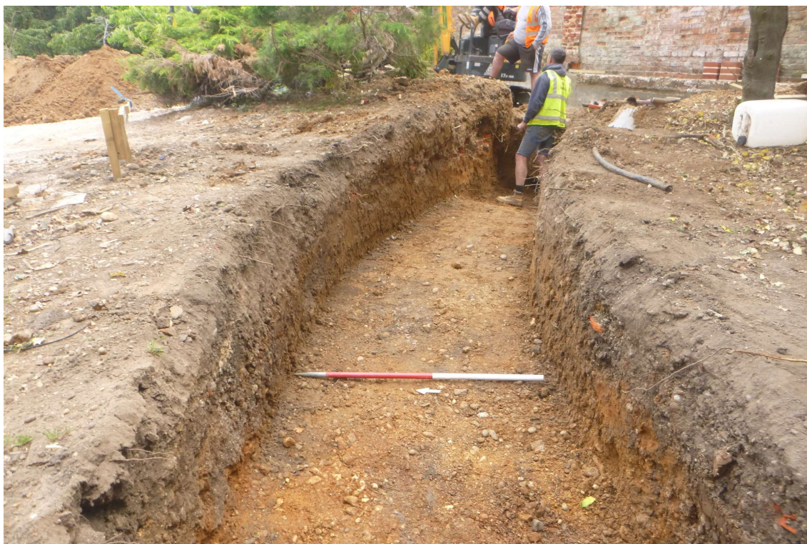
Photograph 6 Trench connecting the new plant room to the house, looking north-east.
