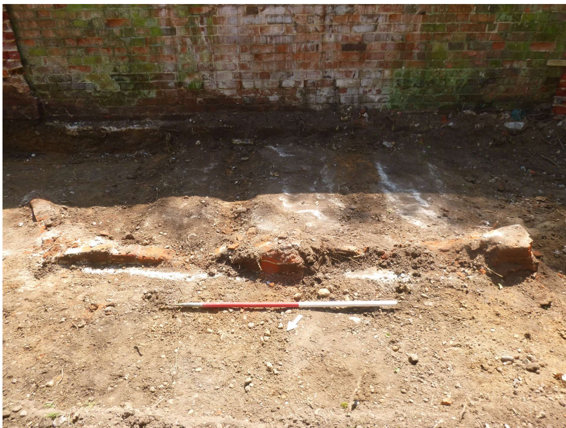
Photograph 4 Close-up of brick and concrete foundations, looking south-east.
