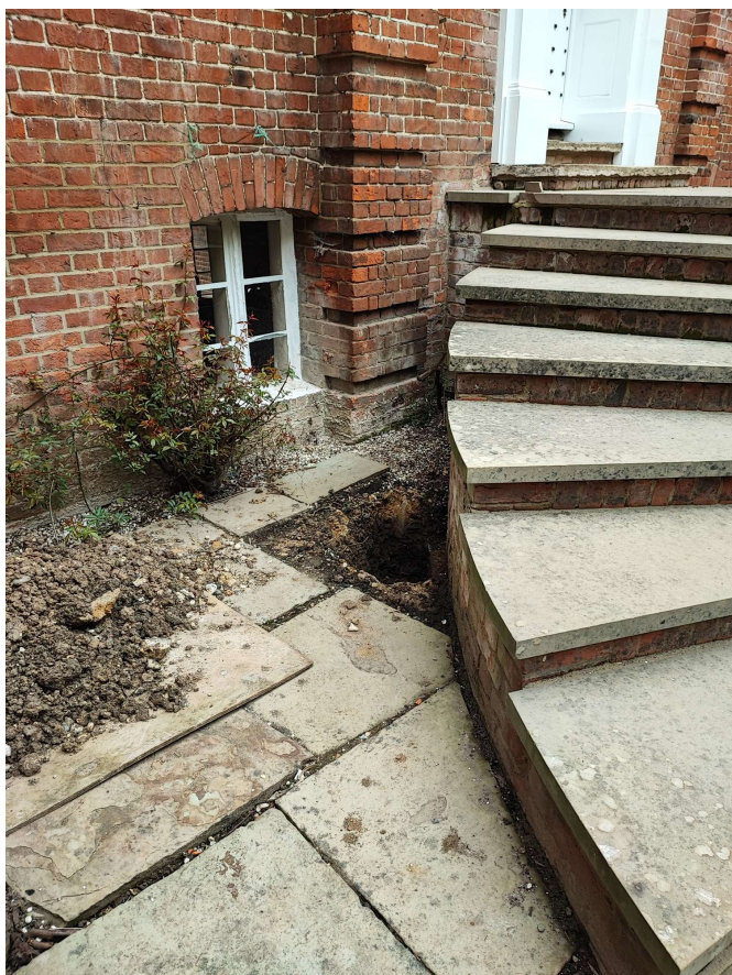
Photograph 1 Trial-pit 2 to south-west of front stairs, looking north-east.
