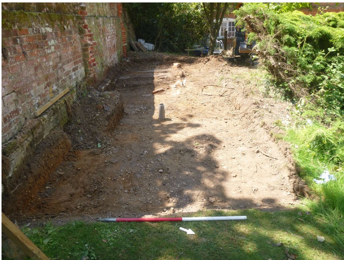
Photograph 3 Ground reduction area along boundary wall, looking south-west.
