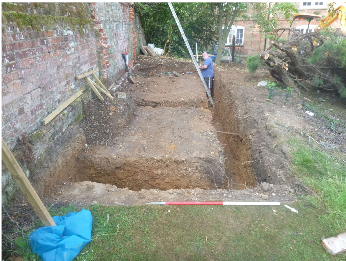
Photograph 5 Foundation trenches within ground reduction area, looking south-west.
