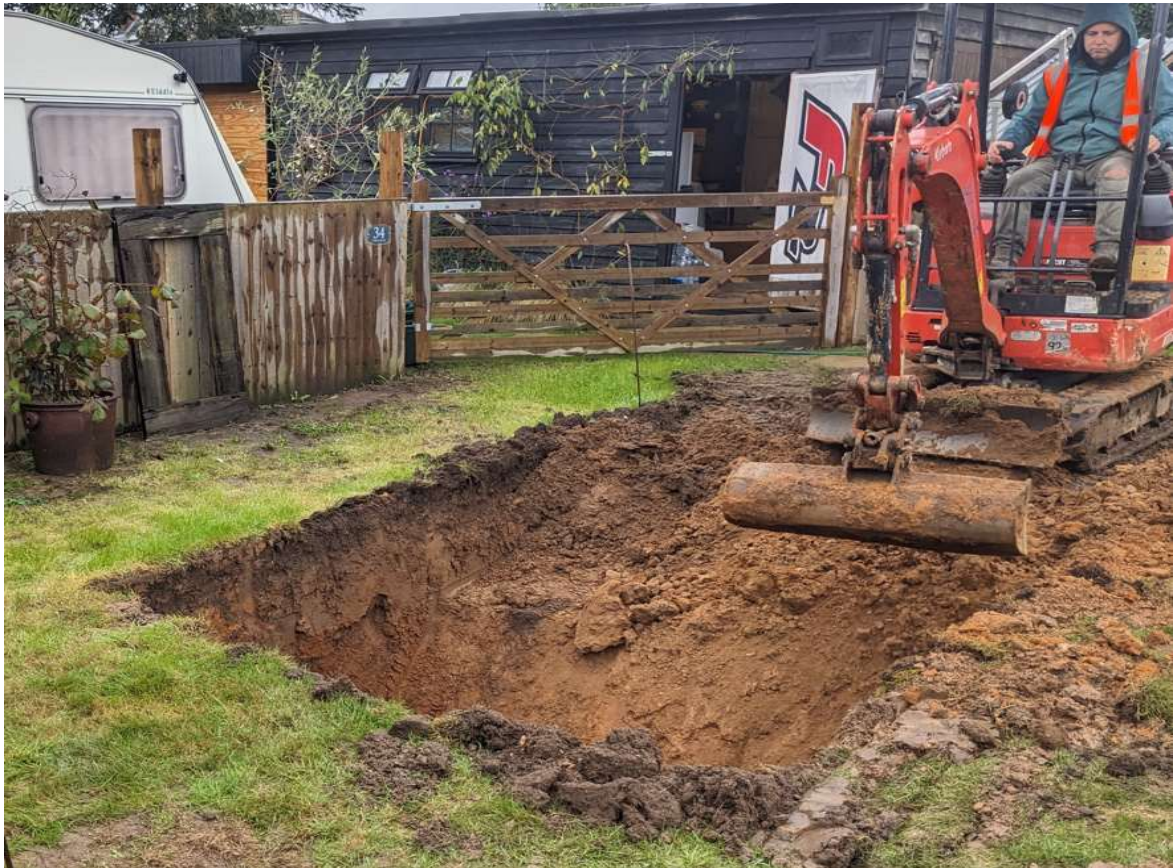
Photograph 3 Soakaway during excavation, view south-west.
