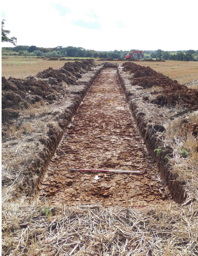
Photograph 2 T8 trench shot – looking south
