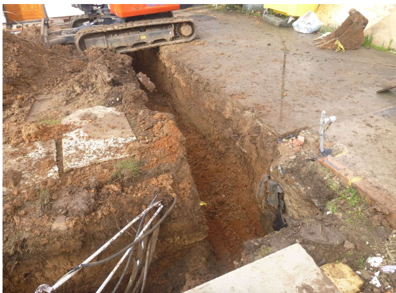
Photograph 3 Foundation trenching – looking north-west
