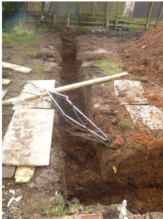
Photograph 2 Foundation trenching – looking south
