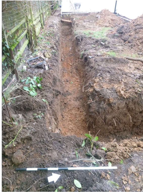
Photograph 1 Foundation trenching – looking west north-west
