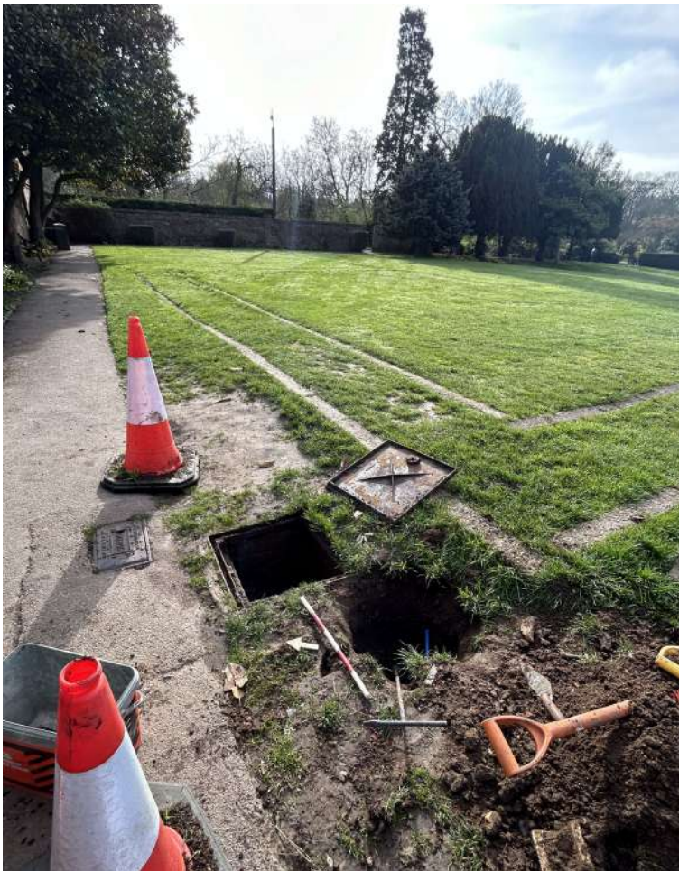
Photograph 4 Location shot of inspection chamber and excavated hole, view east.
