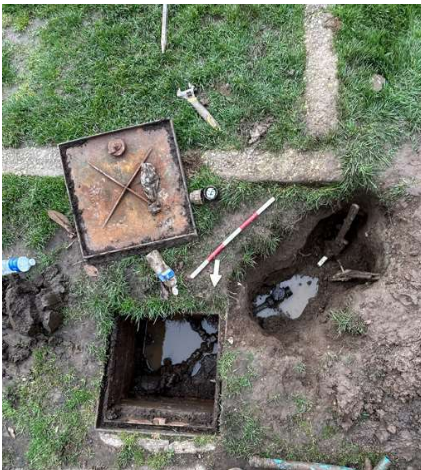
Photograph 1 Plan view of inspection chamber and excavated hole, view south.
