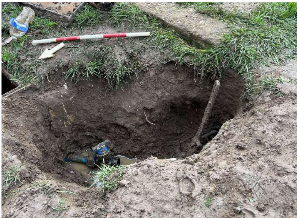
Photograph 2 North-west facing section of excavated hole, view south-east.
