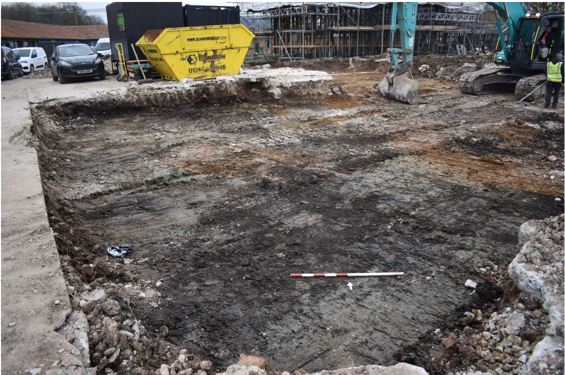
Photograph 11 The stripped footprint of the new extension south-west of the Bailey Barn, view north.
