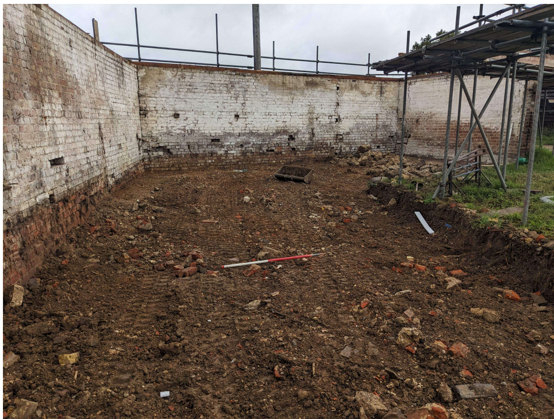
Photograph 1 The stripped footprint of Pond Barn, view north-west.
