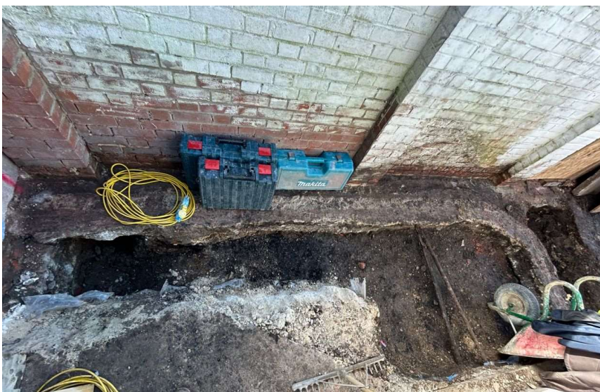
Photograph 2 General shot of completed trench within south area, view south-west.
