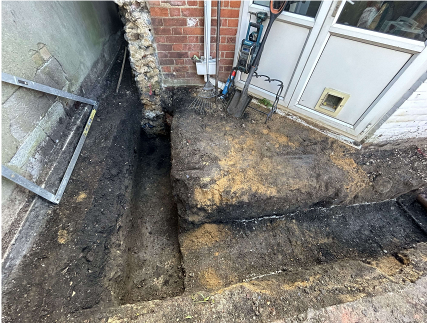
Photograph 3 Northern area of trenching, view east.
