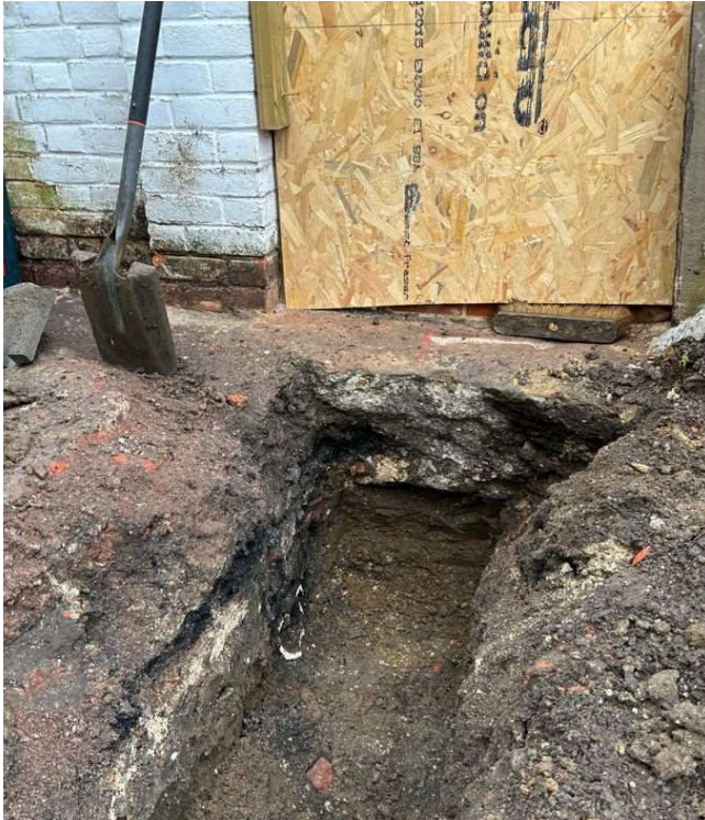
Photograph 7 View of gate (boarded up) and F2, view south.
