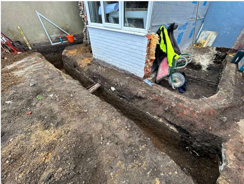
Photograph 1 General shot of completed trenches, view north-east.
