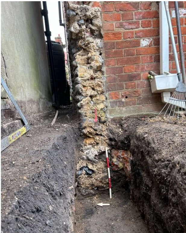
Photograph 4 East side of F1, view east.
