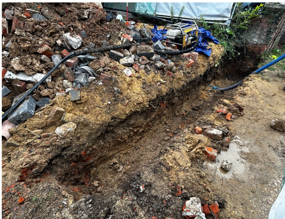
Photograph 11 Working shot of foundations for new wall. View south.
