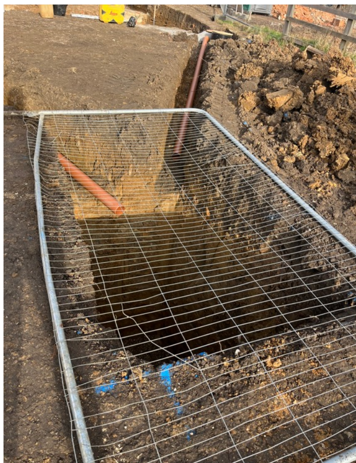
Photograph 7 Soakaway 1 and associated drainage. View north-west.
