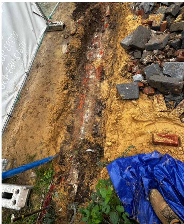
Photograph 12 A section of an old wall foundation prior to removal. View north-east.
