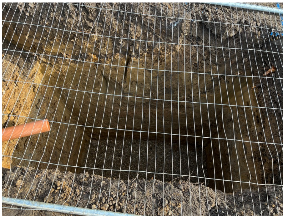
Photograph 8 Soakaway 1. View east.
