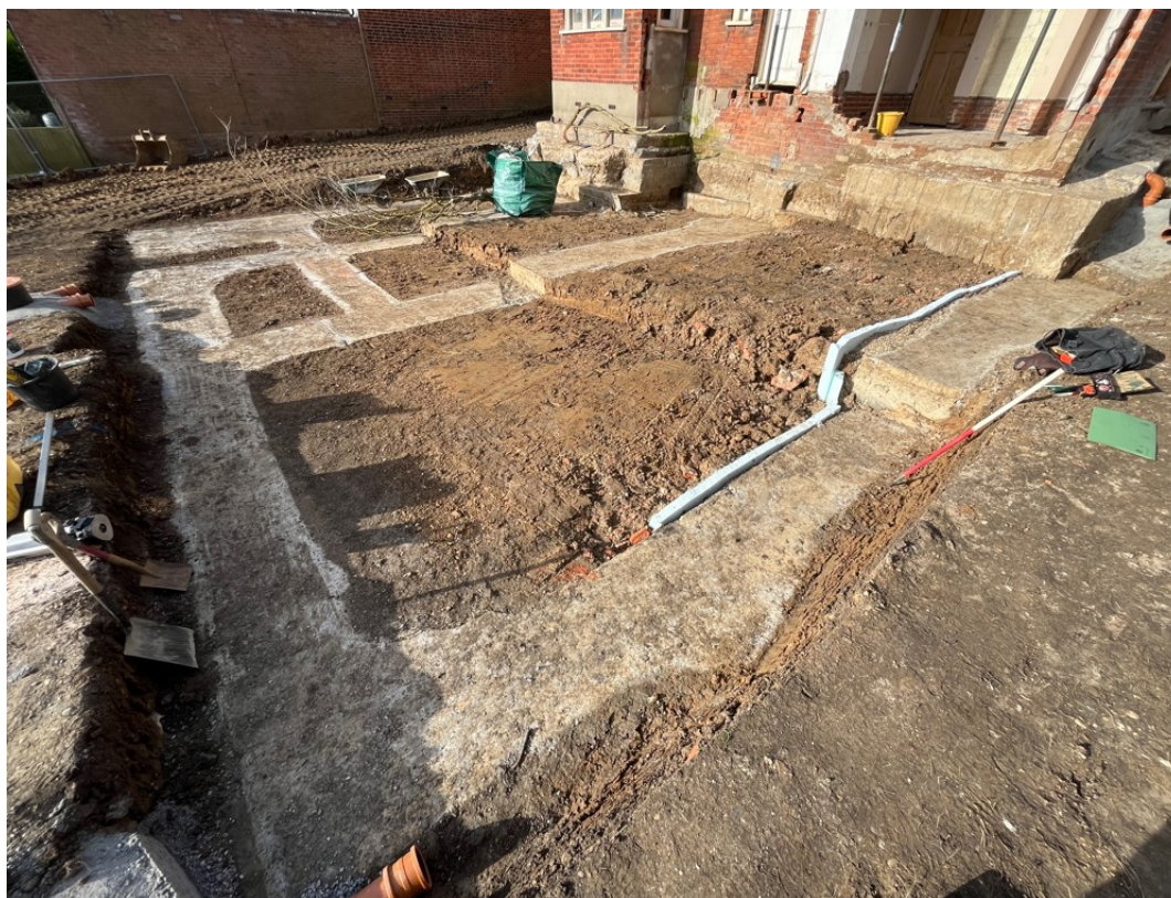
Photograph 5 Completed rear extension foundations. View west.
