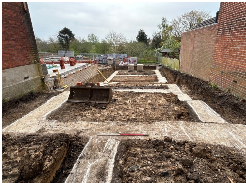
Photograph 2 New dwelling foundations from north-west end. View south-east.
