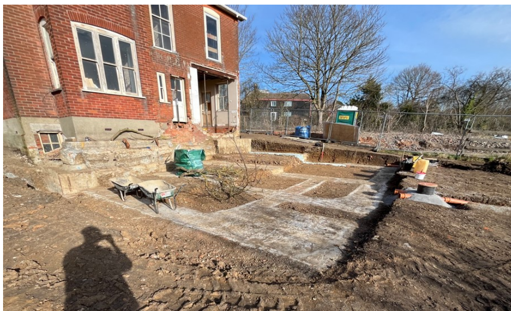
Photograph 6 Completed rear extension foundations. View east.
