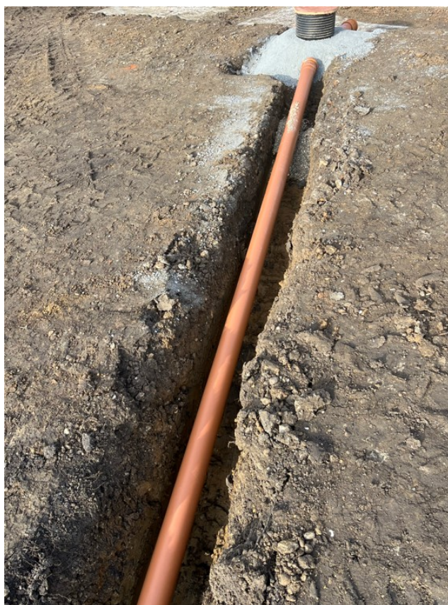
Photograph 9 Associated drainage between soakaway 1 and rear extension. View north-west.
