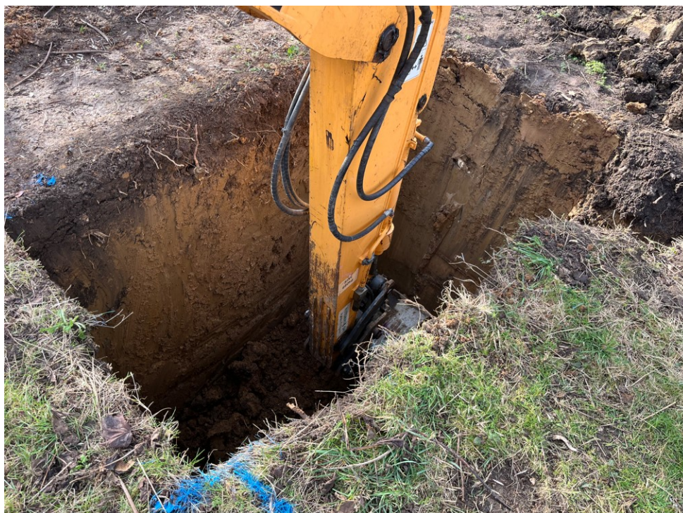
Photograph 10 Working shot of soakaway 2. View south.
