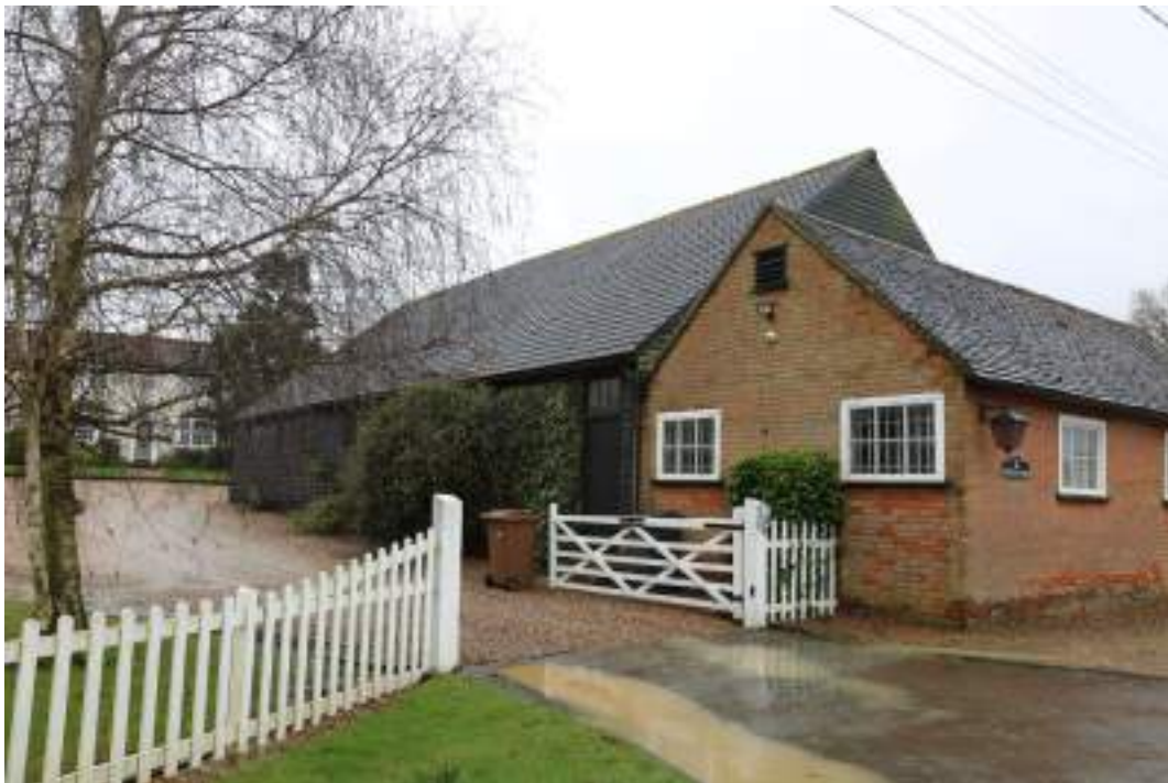
MGWF24_PhotoGraph_183 Eastern elevation of building 2. Photograph taken facing south-west.
