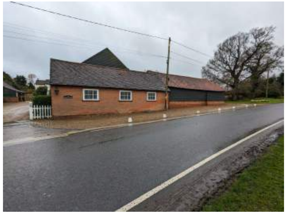
MGWF24_PhotoGraph_198 Northern elevation of building 2. Photograph taken facing south.
