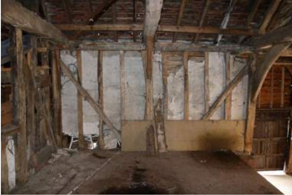
Photograph 13 Western wall of bay 4 of threshing barn. Photograph taken facing west.
