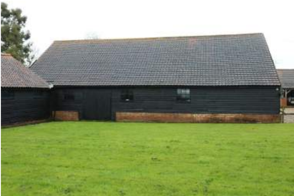
Photograph 29 Western elevation of building 2. Photograph taken facing east.
