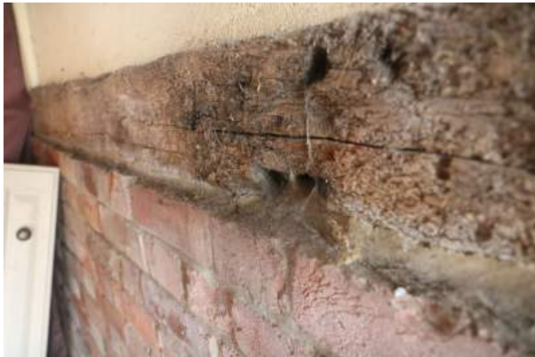
MGWF24_PhotoGraph_100 Interior detail shot of reused timber sill-beam in carport. Photograph taken facing south-east.
