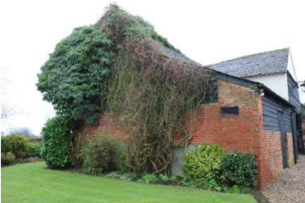
Photograph 3 Northern elevation of building 1. Photograph taken facing south-east.
