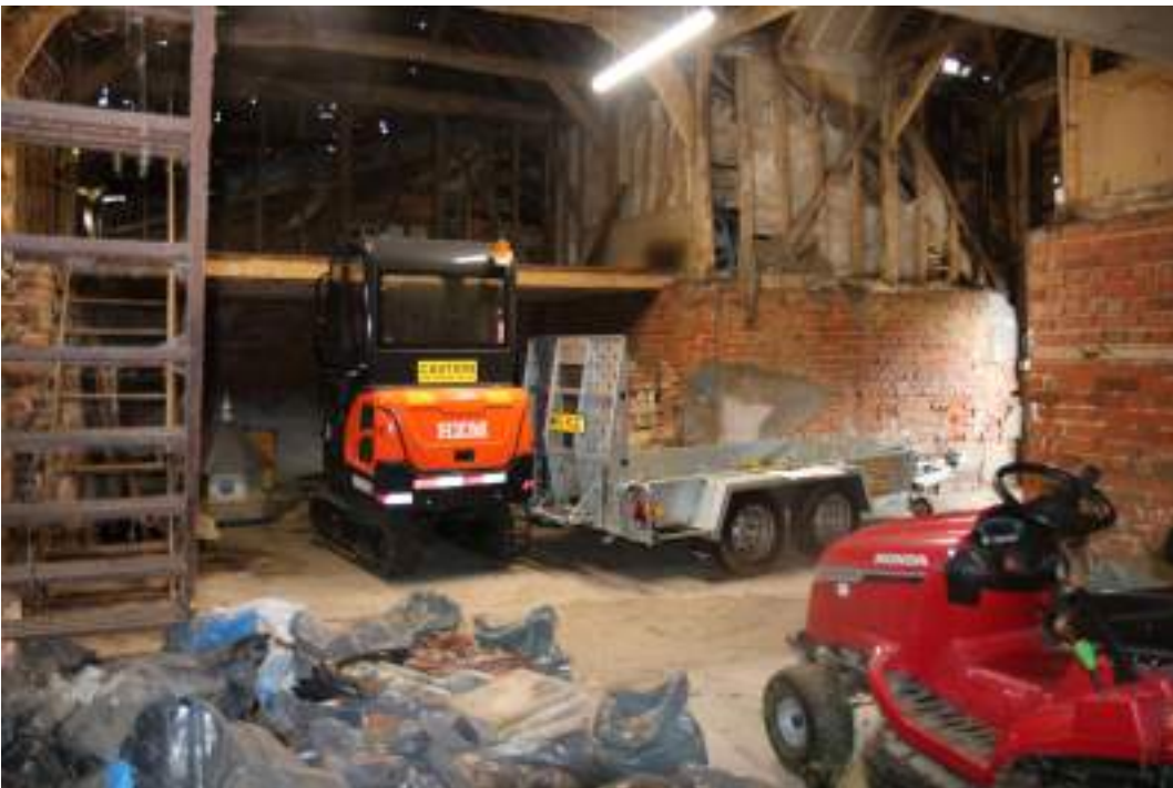
MGWF24_PhotoGraph_103 Interior shot of threshing barn. Photograph taken facing south-west.
