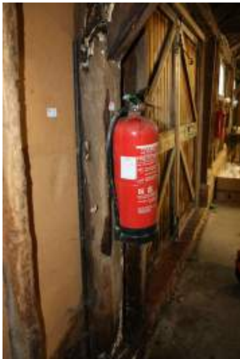
MGWF24_Phograph_063 Interior detail shot of reused timber intermediate post between bays 4 and 5, small barn. Photograph taken facing south-west.
