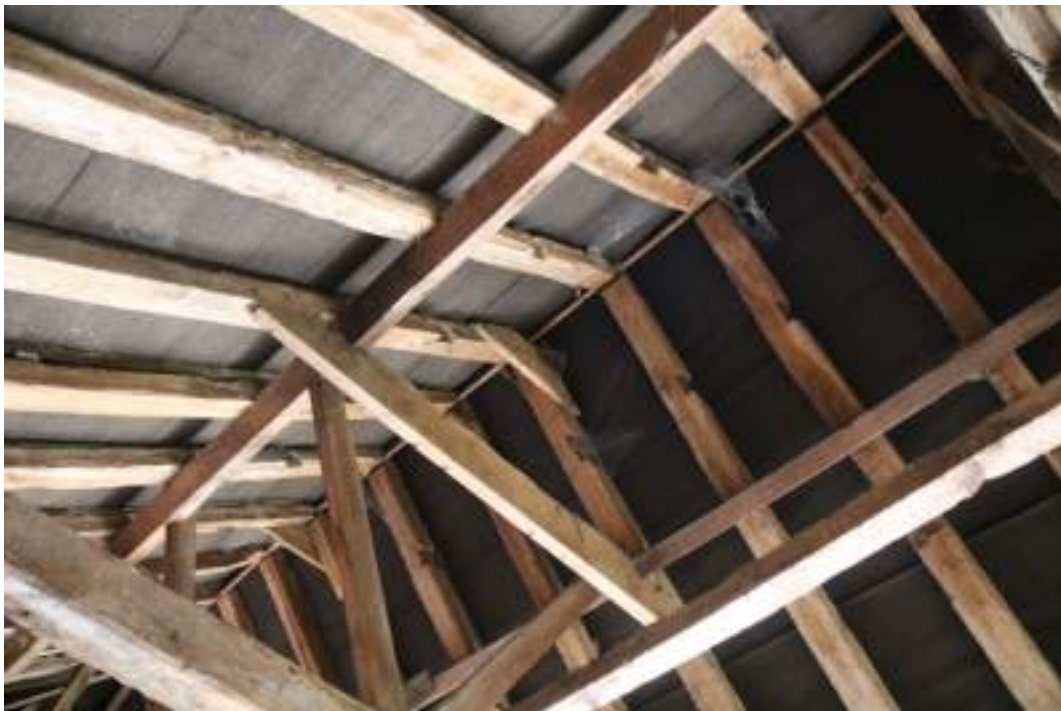
MGWF24_PhotoGraph_099 Interior detail shot of reused timbers of rafters in carport. Photograph taken facing south-west.
