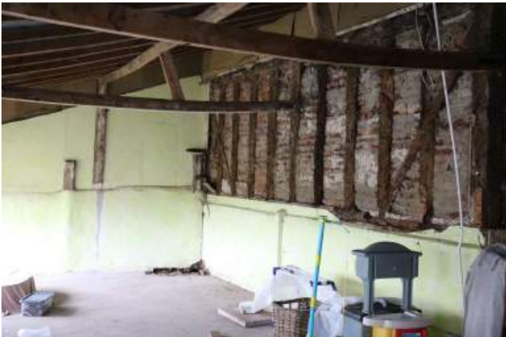
Photograph 21 Interior of lean-to 3. Photograph taken facing south-west.
