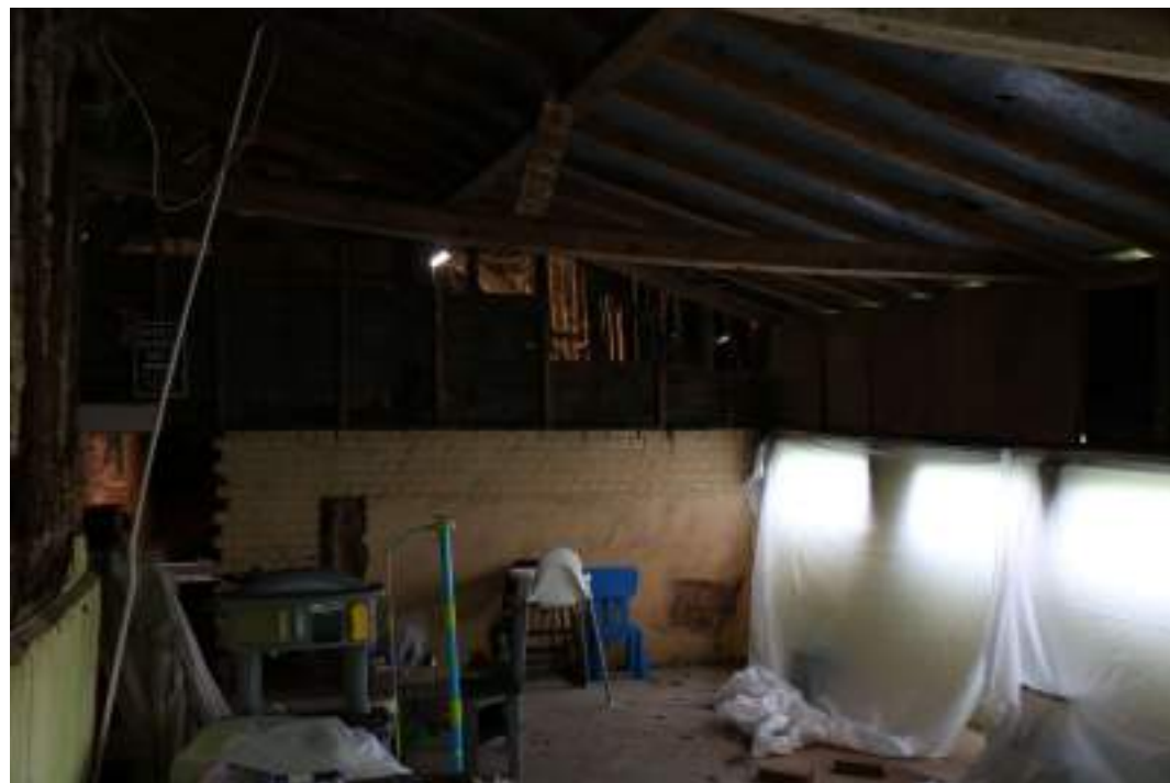
MGWF24_PhotoGraph_160 Interior shot of lean-to 3. Photograph taken facing north.
