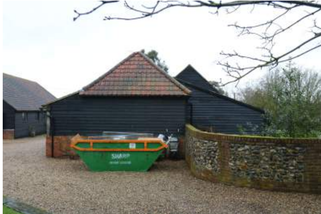
MGWF24_PhotoGraph_180 Southern elevation of building 1. Photograph taken facing north.
