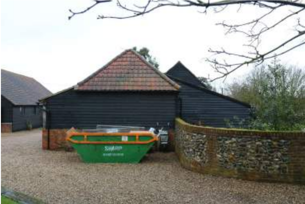
Photograph 6 Southern elevation of building 1. Photograph taken facing north.
