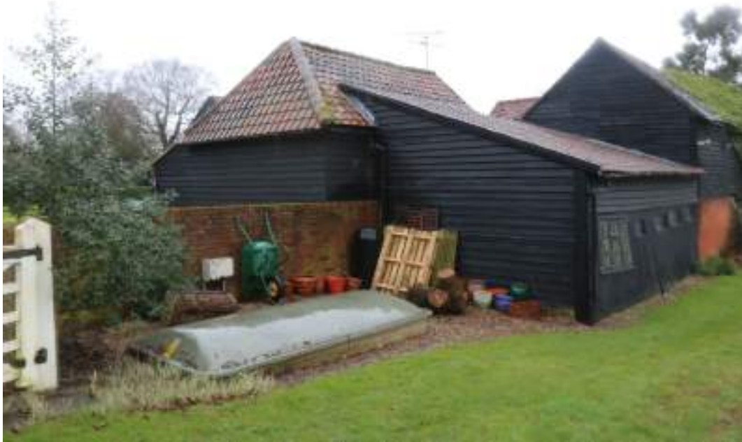
MGWF24_PhotoGraph_181 Southern elevation of building 1. Photograph taken facing north-west.
