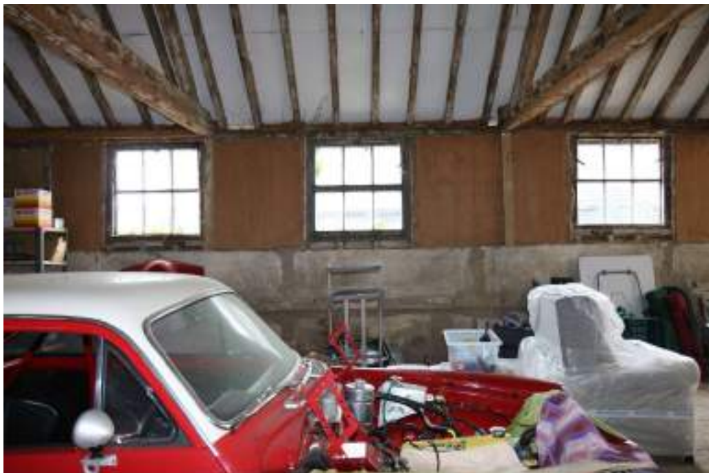
Photograph 34 Interior of cowshed, bay 4. Photograph taken facing east.
