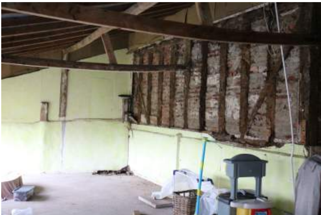
MGWF24_PhotoGraph_159 Interior shot of lean-to 3. Photograph taken facing south-west.
