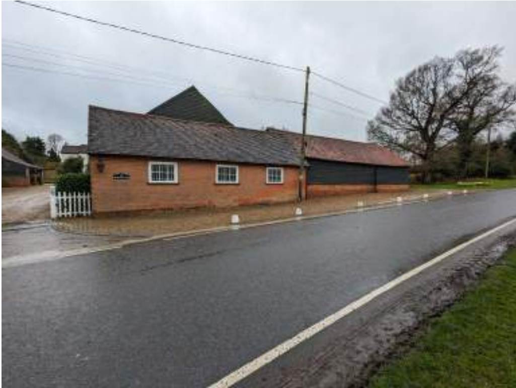
Photograph 30 Northern elevation of building 2. Photograph taken facing south.
