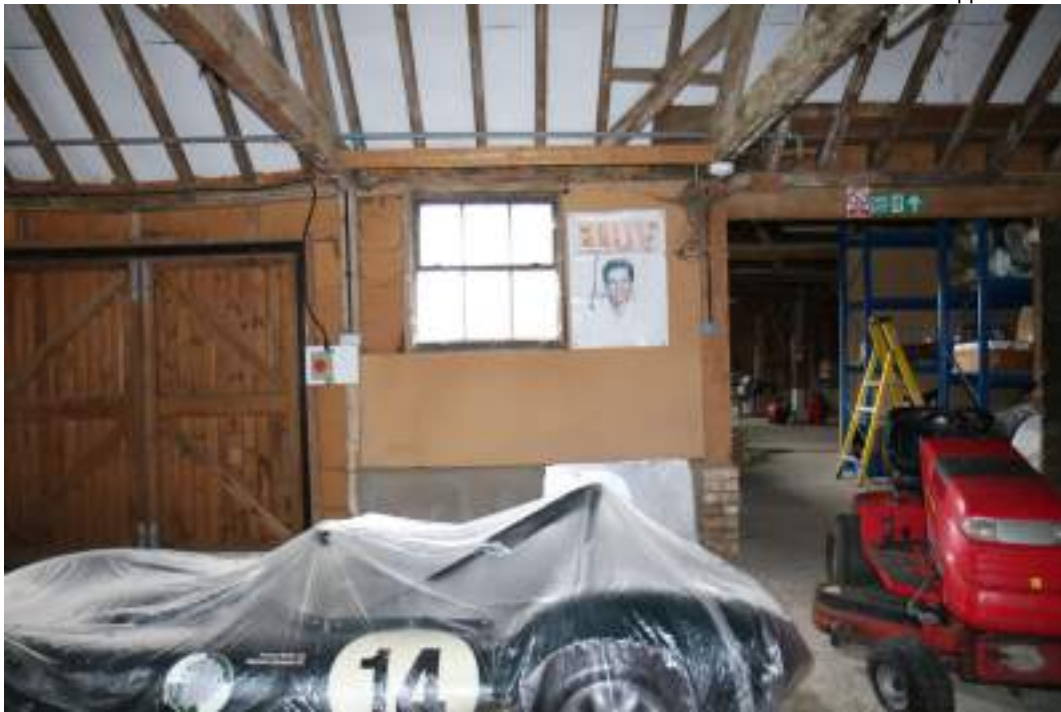
MGWF24_PhotoGraph_021 Interior shot of cowshed, bay 6. Photograph taken facing west.
