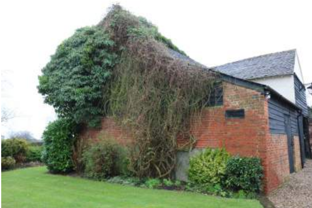
MGWF24_PhotoGraph_179 Northern elevation of building 1. Photograph taken facing south-east.
