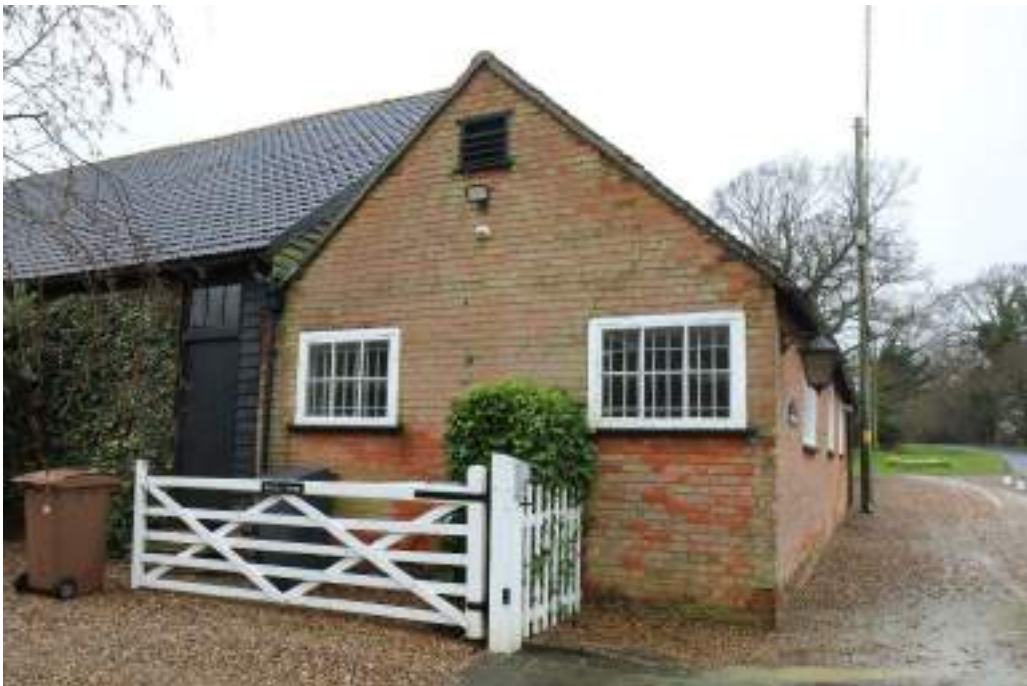
Photograph 27 Eastern elevation of brick building. Photograph taken facing south-west.
