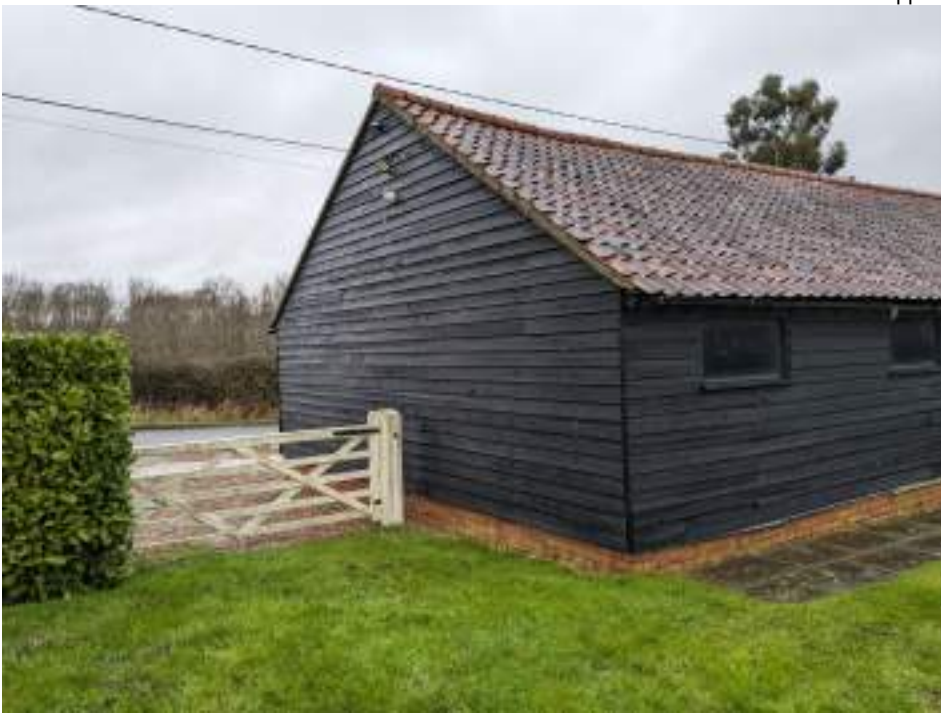
MGWF24_PhotoGraph_193 Western elevation of building 2. Photograph taken facing north-east.
