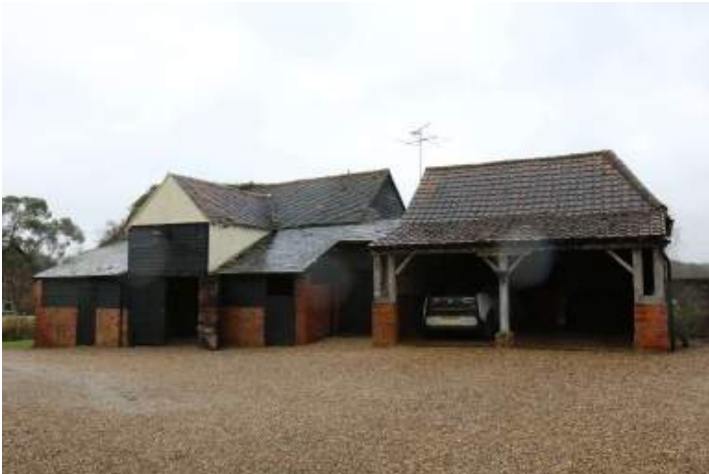
Photograph 1 Western elevation of building 1. Photograph taken facing north-east.
