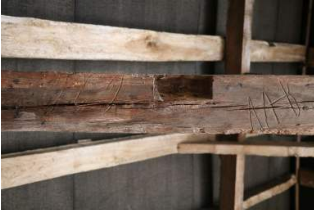
Photograph 25 Detail of reused tie-beam, with Baltic timber mark, in carpenter.
