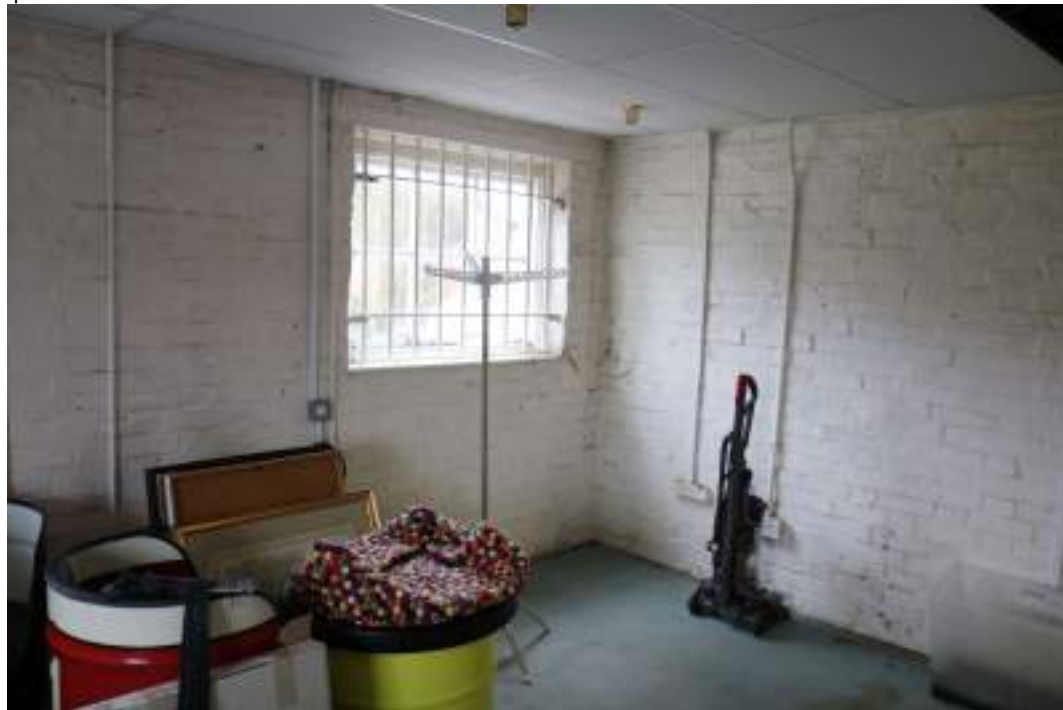
MGWF24_PhotoGraph_034 Interior shot of brick building, room 2. Photograph taken facing north-east.
