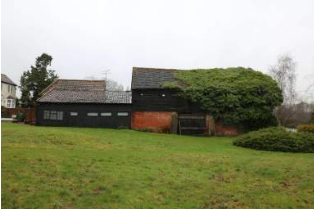
Photograph 4 Eastern elevation of building 1. Photograph taken facing west.
