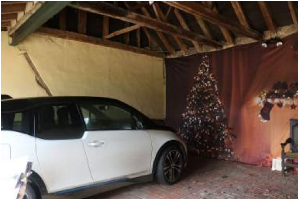
Photograph 22 Interior of carport. Photograph taken facing north-east.
