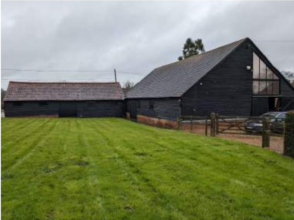
Photograph 28 Southern elevation of building 2. Photograph taken facing north.
