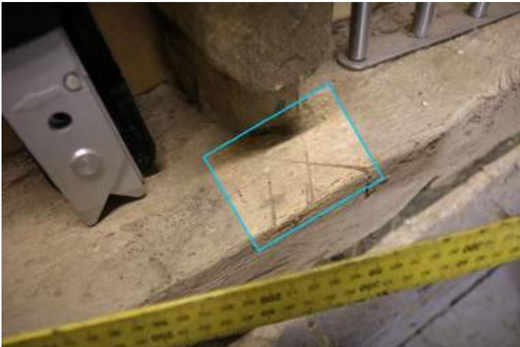
Photograph 42 Detail of cubic volume mark on sill-beam in small barn. Photograph taken facing north-west.
