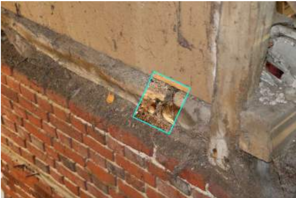
Photograph 12 Detail of scarf-joint in bay 4 of threshing barn. Photograph taken facing south-west.
