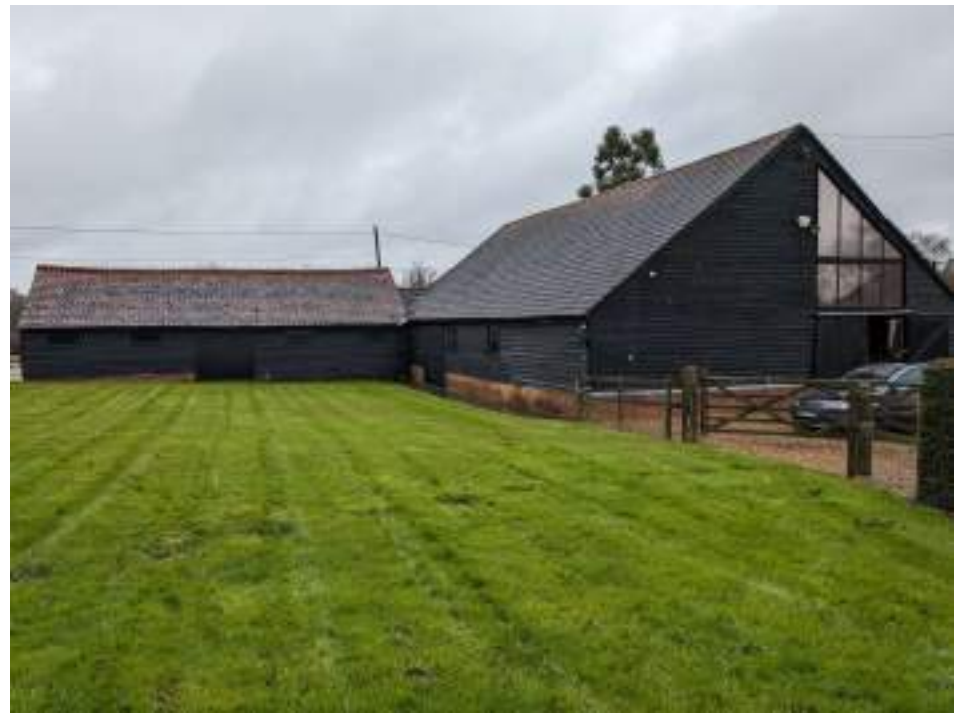
MGWF24_PhotoGraph_194 Southern elevation of building 2. Photograph taken facing north.
