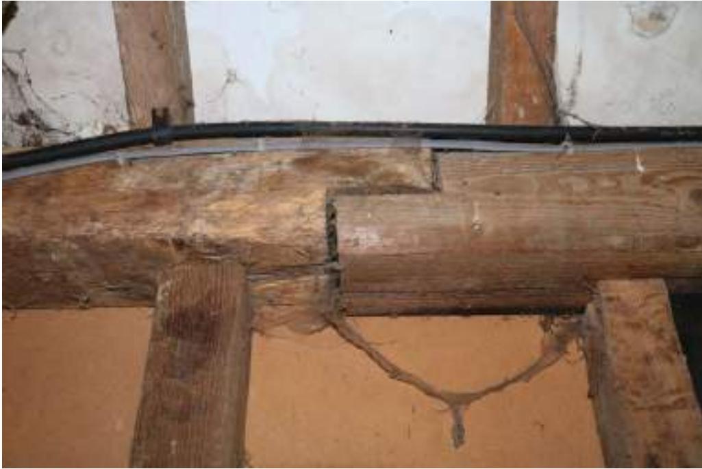
Photograph 45 Detail of scarf-joint in wall-plate of bay 5 of the small barn. Photograph taken facing south.
