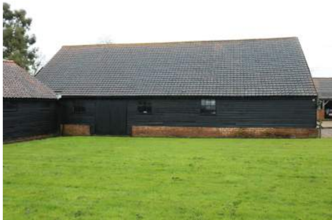
MGWF24_PhotoGraph_188 Western elevation of building 2 (cowshed). Photograph taken facing East.
