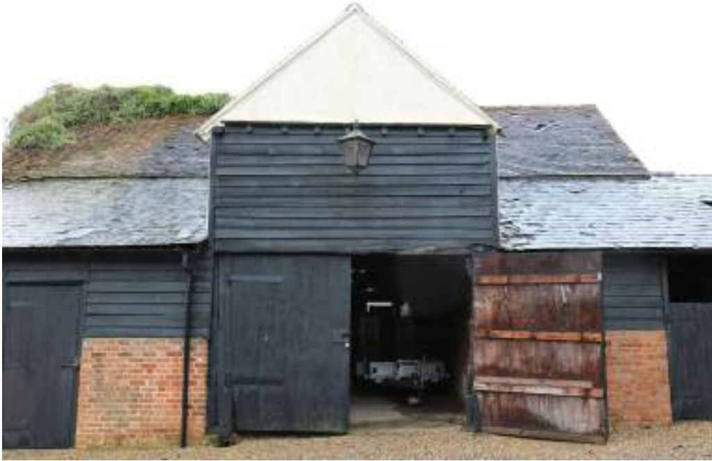
Photograph 2 Detail of barn doors on western elevation of threshing barn. Photograph taken facing east.
