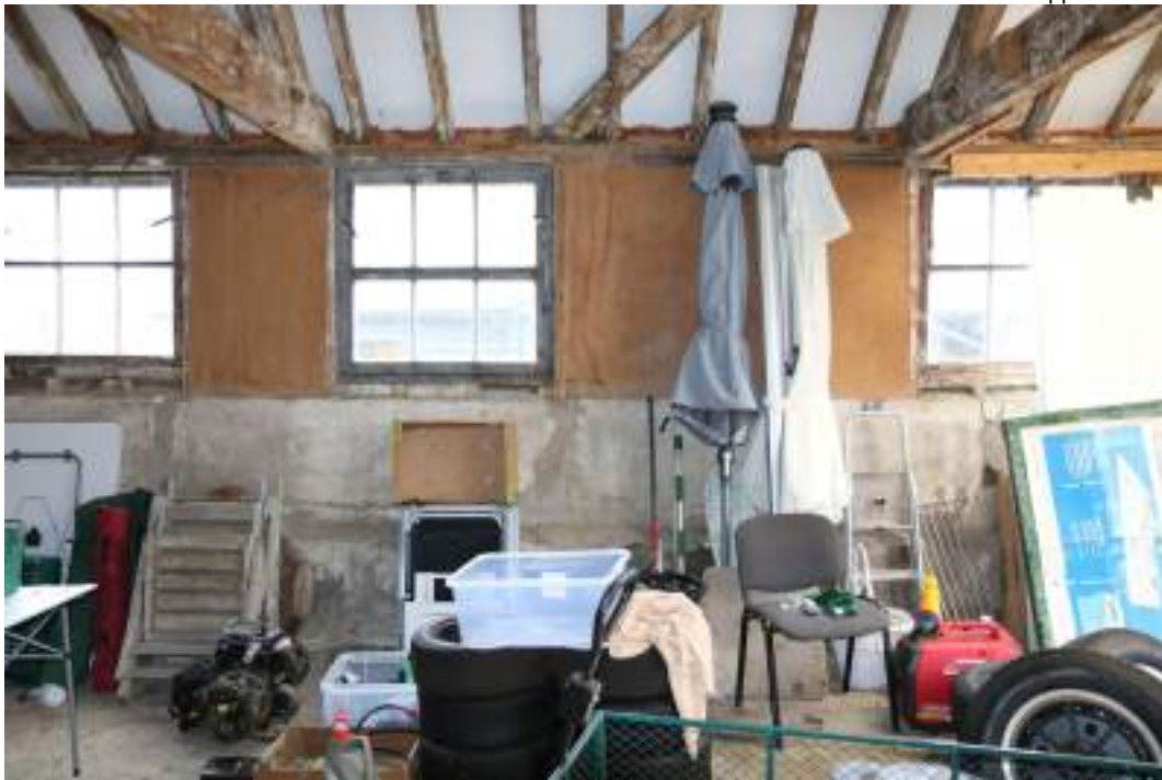
MGWF24_PhotoGraph_009 Interior shot of cowshed, bay 2. Photograph taken facing east.
