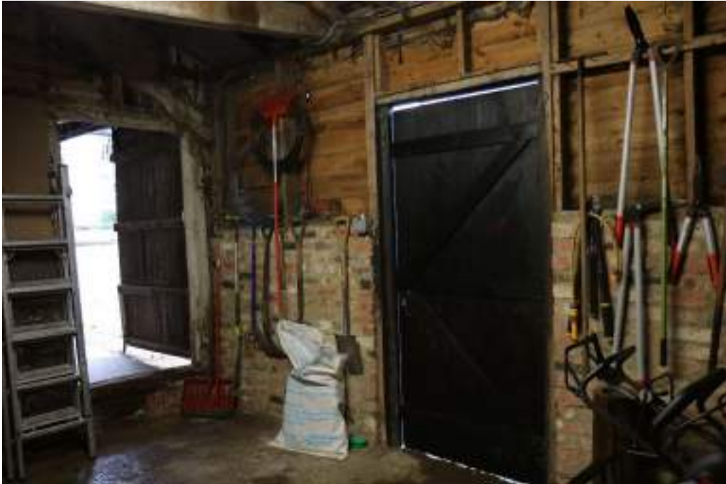
Photograph 17 Interior of lean-to 3. Photograph taken facing south-west.
