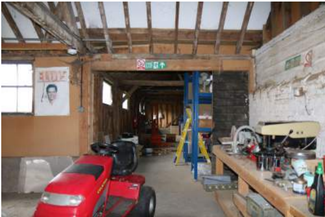
MGWF24_PhotoGraph_023 Interior shot of cowshed, bay 7. Photograph taken facing west.
