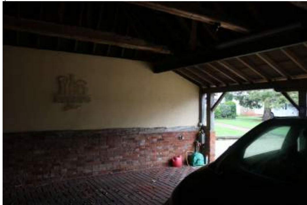
MGWF24_PhotoGraph_090 Interior shot of carport. Photograph taken facing south-west.
