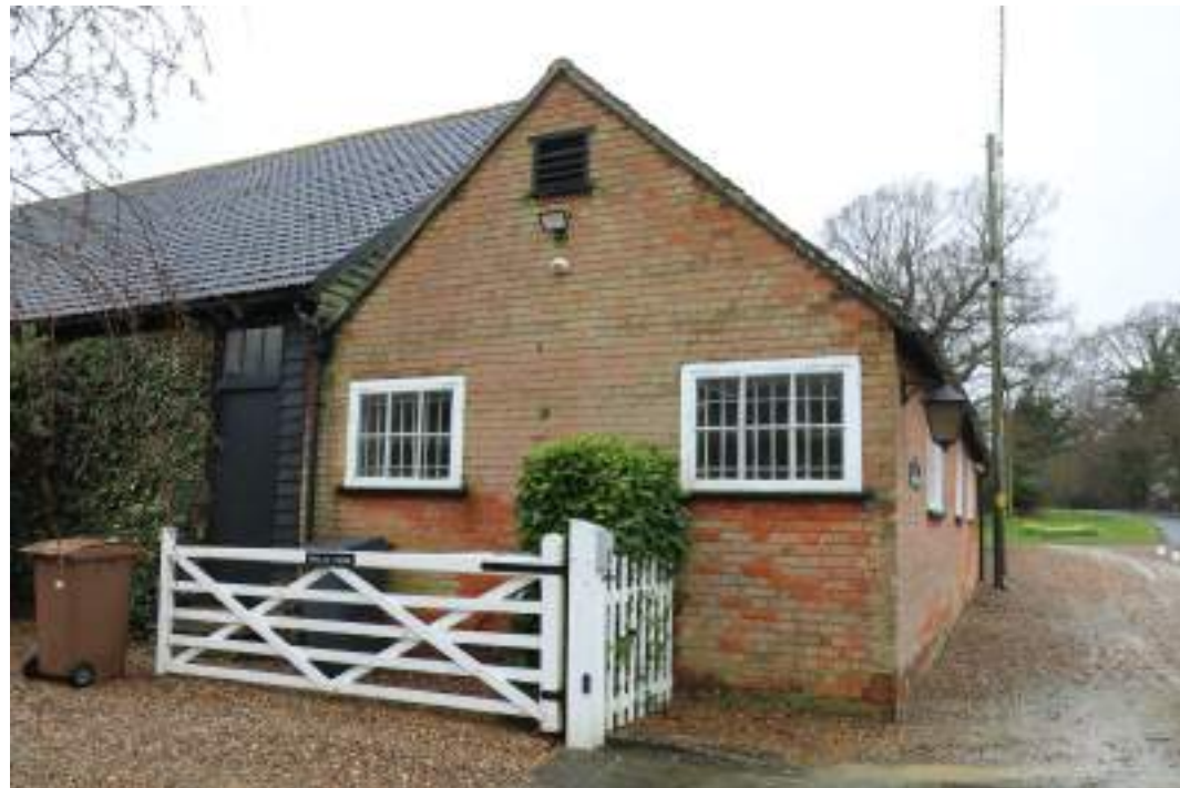
MGWF24_PhotoGraph_184 Detail shot of windows on eastern elevation of brick building. Photograph taken facing south-west.
