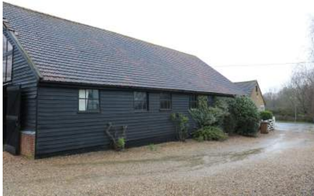
MGWF24_PhotoGraph_182 Eastern elevation of building 2. Photograph taken facing north-west.
