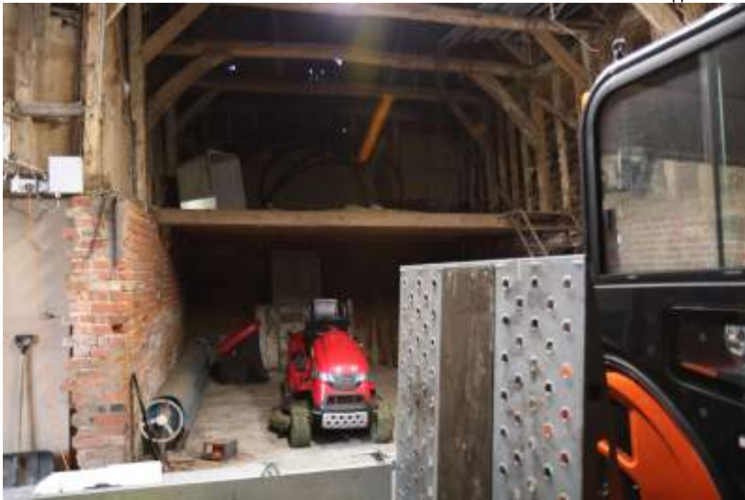
MGWF24_Phograph_105 Interior shot of threshing barn. Photograph taken facing north-east.
