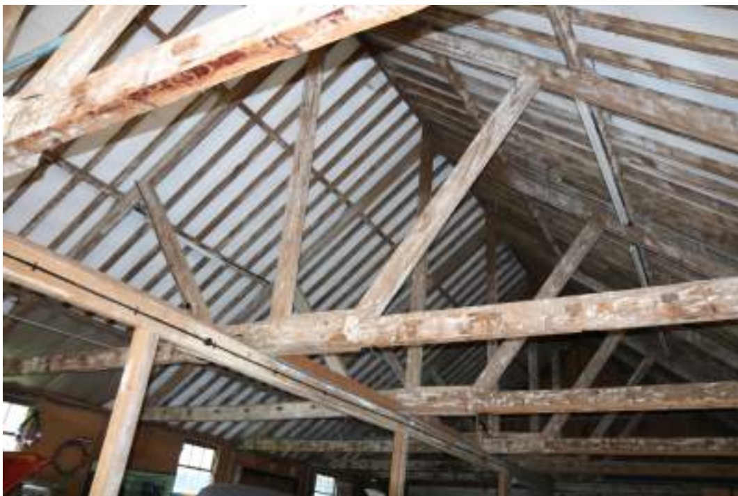
MGWF24_Phograph_003 Interior shot of cowshed roof construction. Photograph taken facing north-west.
