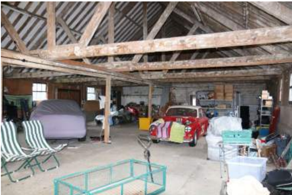
Photograph 31 Interior of cowshed. Photograph taken facing north-west.
