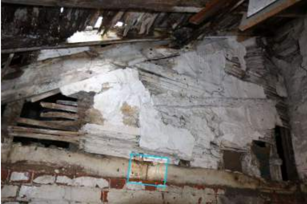
Photograph 19 Interior of lean-to 2, showing lath and plaster wall. Sill-beam scarf-joint and carpenter's marks highlighted in blue. Photograph taken facing north-east.
