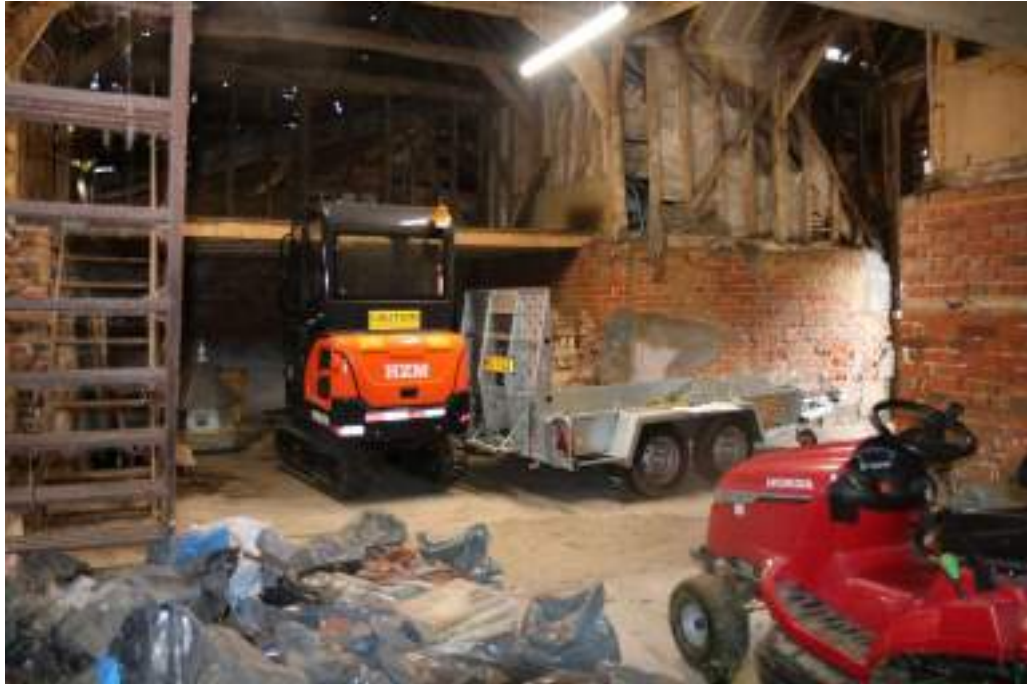
Photograph 8 Interior of threshing barn. Photograph taken facing south-west.
