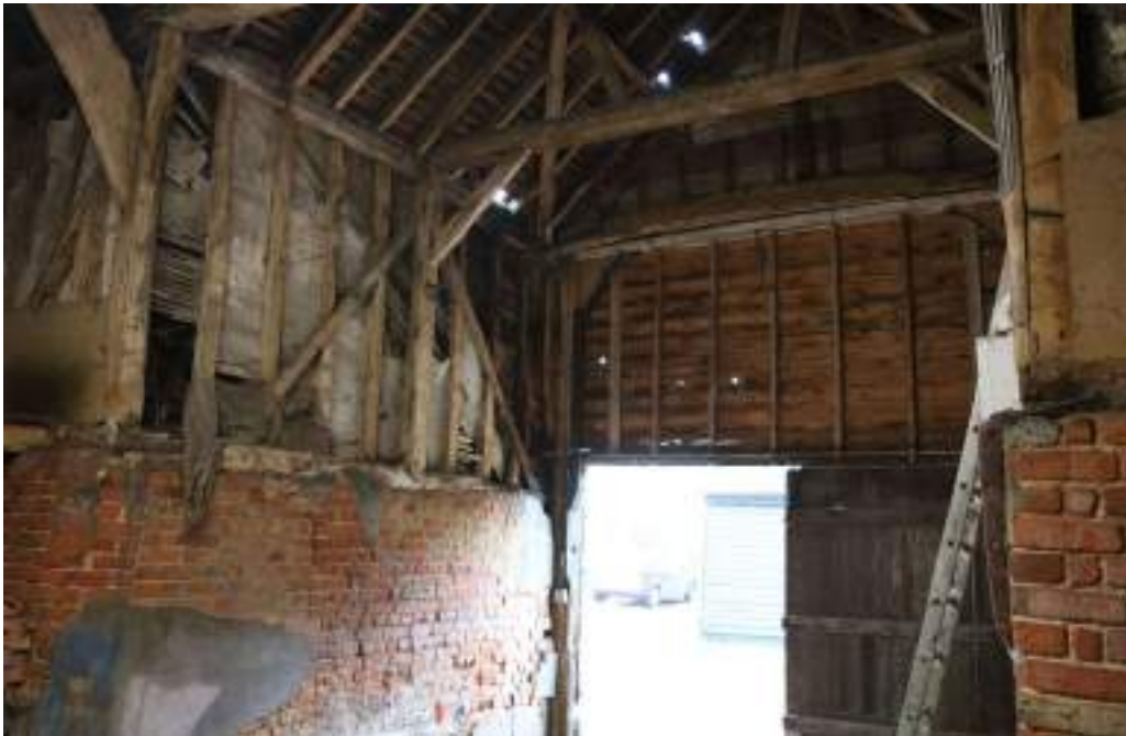
Photograph 14 Interior of midstrey of threshing barn. Photograph taken facing south-east.
