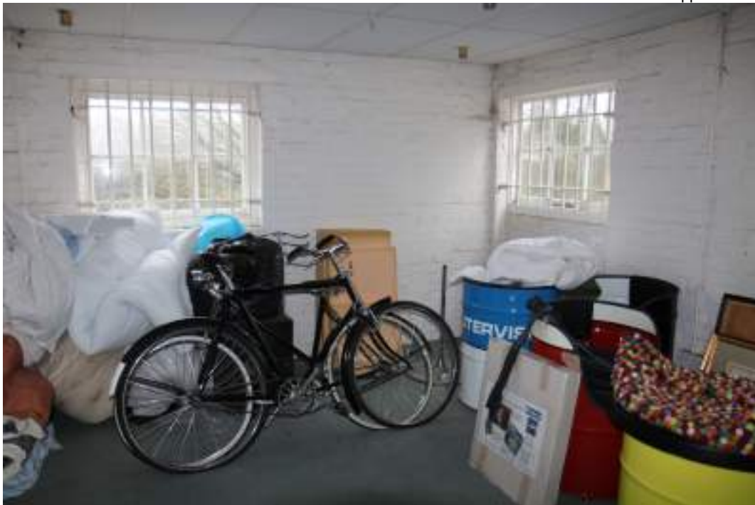
MGWF24_PhotoGraph_033 Interior shot of brick building, room 2. Photograph taken facing north-east.
