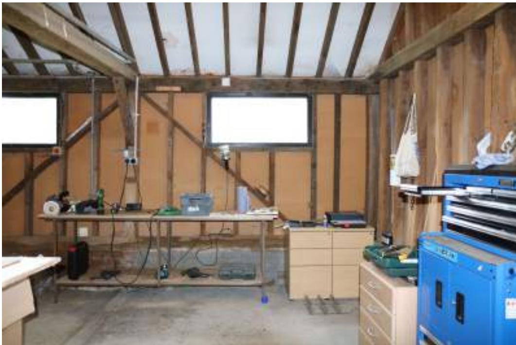
MGWF24_PhotoGraph_039 Interior shot of small barn bay 1. Photograph taken facing south.
