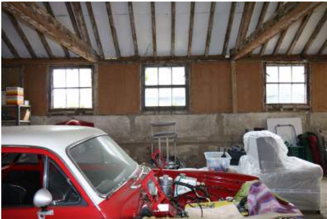
MGWF24_PhotoGraph_015 Interior shot of cowshed, bay 4. Photograph taken facing east.
