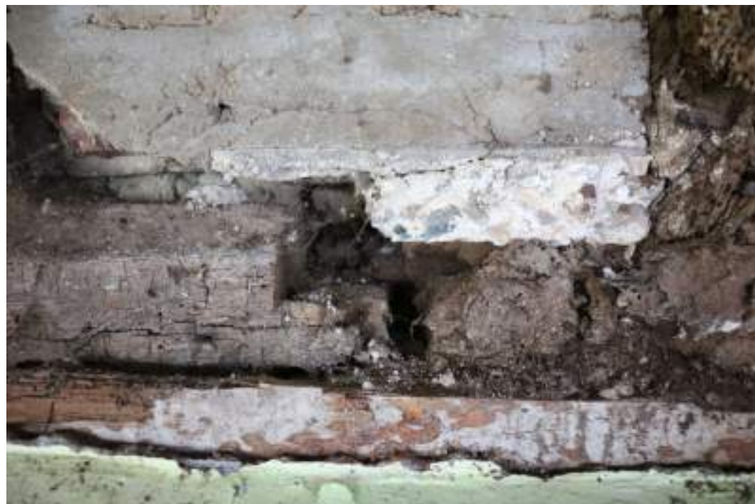
MGWF24_PhotoGraph_164 Interior detail shot of side-halved scarf-joint in sill-beam in lean-to 3. Photograph taken facing north.
