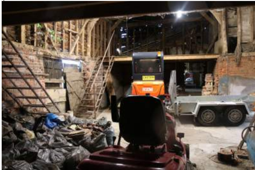
MGWF24_PhotoGraph_102 Interior shot of threshing barn. Photograph taken facing south-east.
