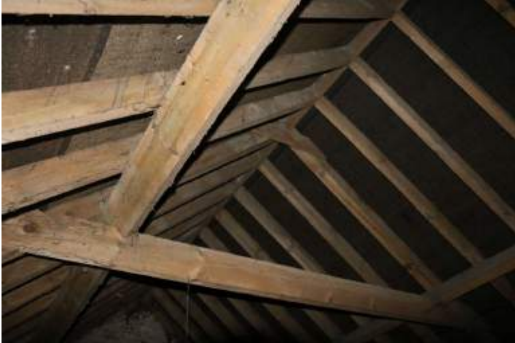
Photograph 36 Detail of roof construction of brick building. Photograph taken facing north-west.
