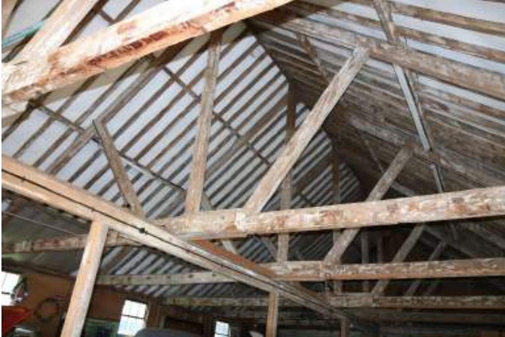
Photograph 32 Detail of cowshed roof construction. Photograph taken facing north-west.
