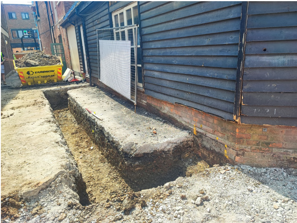
Photograph 5 Side foundation trench, looking south.
