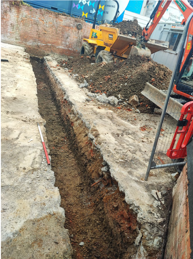
Photograph 4 Rear foundation trench (east side), looking north.
