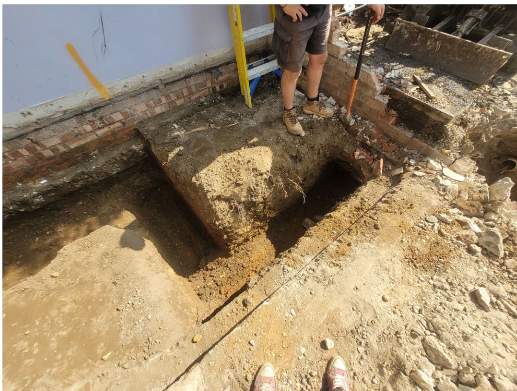
Photograph 2 Foundation trench and ground reduction areas, looking south-east.
