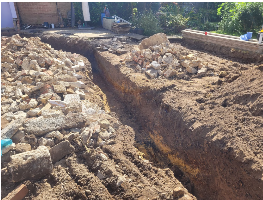
Photograph 1 Foundation trench, also showing ground reduction areas and L3, looking south-east.
