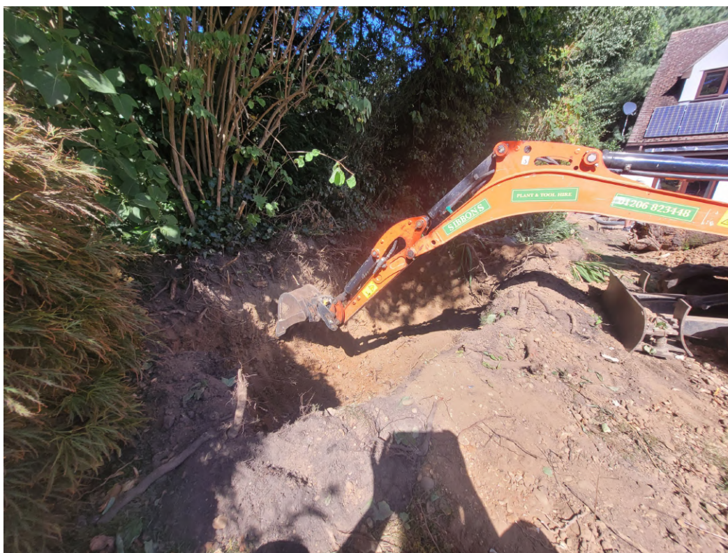
Photograph 4 Excavation of the new soakaway, looking north-north-west.
