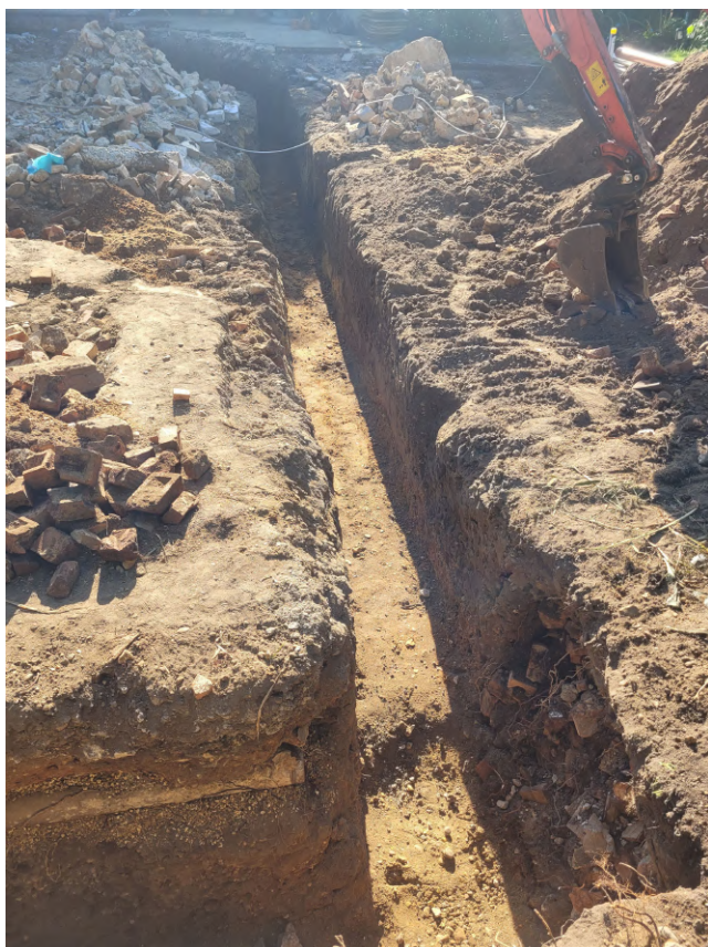
Photograph 3 Foundation trench showing old soakaway and service trench, looking south-east.
