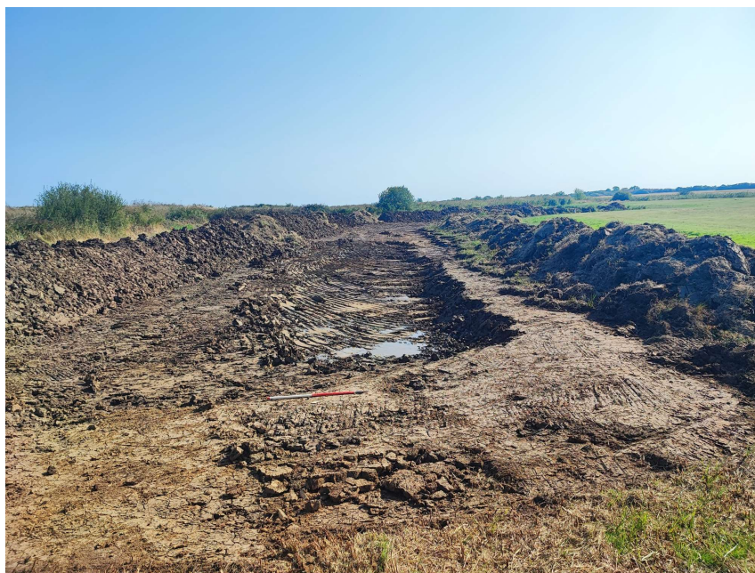
Photograph 1 Stripped area, looking east south-east
