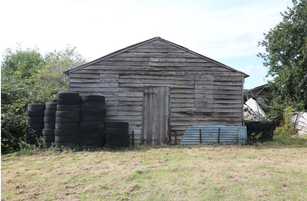
Photograph 39 Eastern elevation of building 21. Photograph taken facing west.
