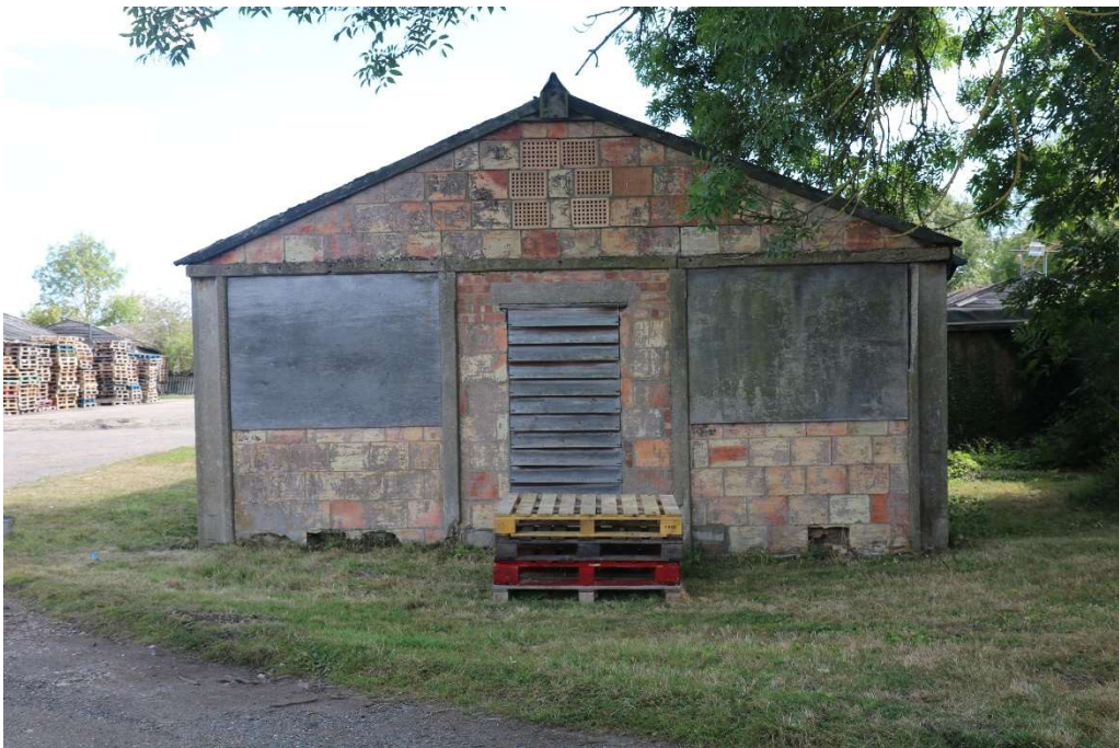
Photograph 9 Western elevation of building 4. Photograph taken facing east.
