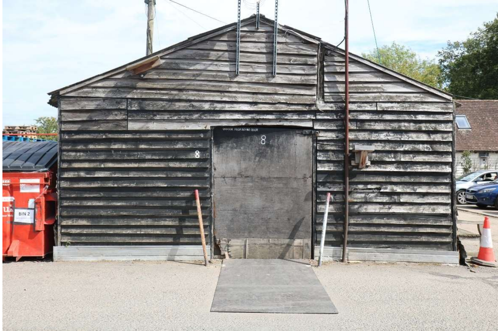
Photograph 20 Western elevation of building 8. Photograph taken facing east.
