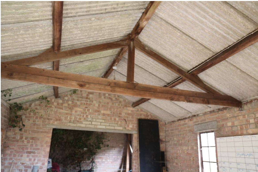
Photograph 17 Detail of roof construction of building 6. Photograph taken facing south-east.
