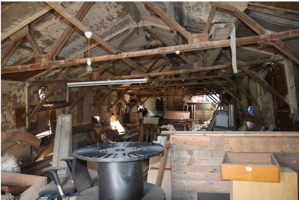
Photograph 33 Interior of building 16. Photograph taken facing south-west.
