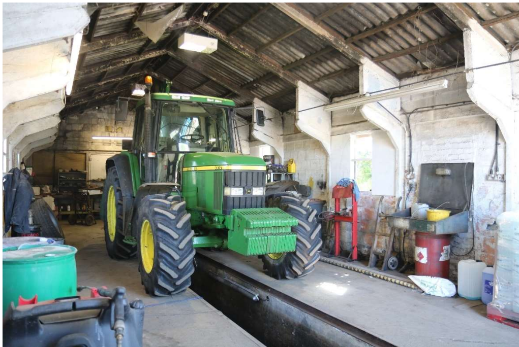
Photograph 13 Interior of building 5. Photograph taken facing south-east.
