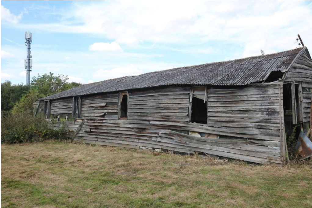
Photograph 18 Southern elevation of building 7. Photograph taken facing north-west.
