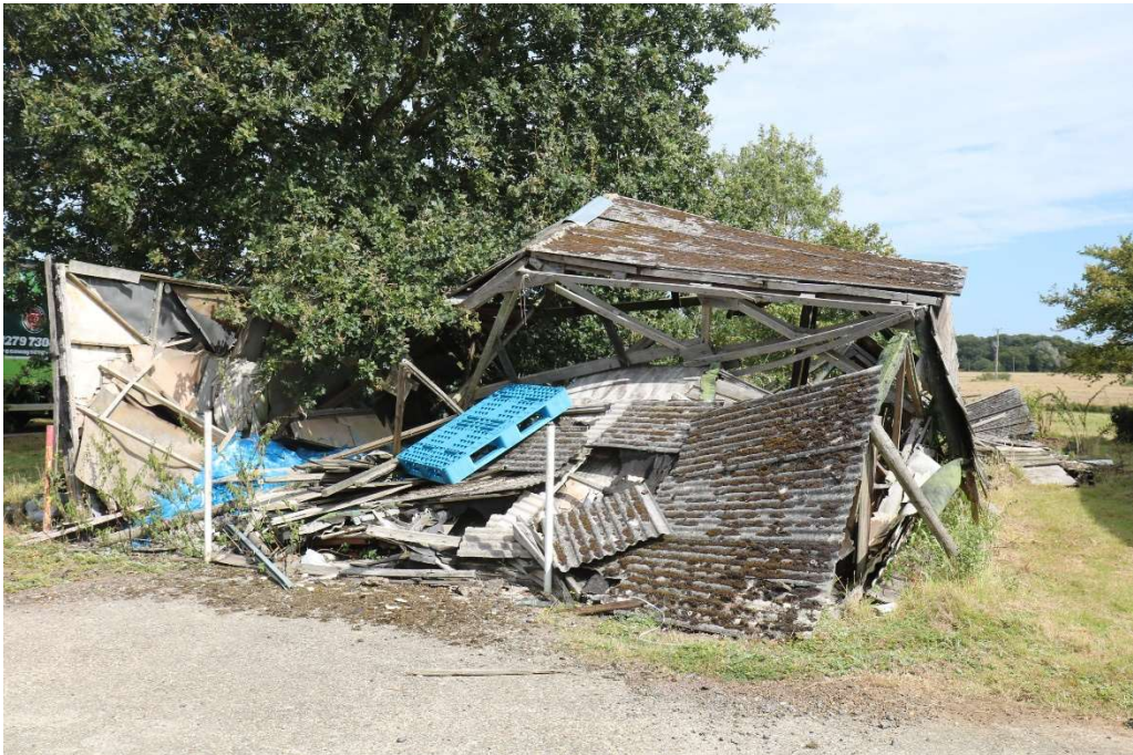
Photograph 38 Building 20. Photograph taken facing south-west.
