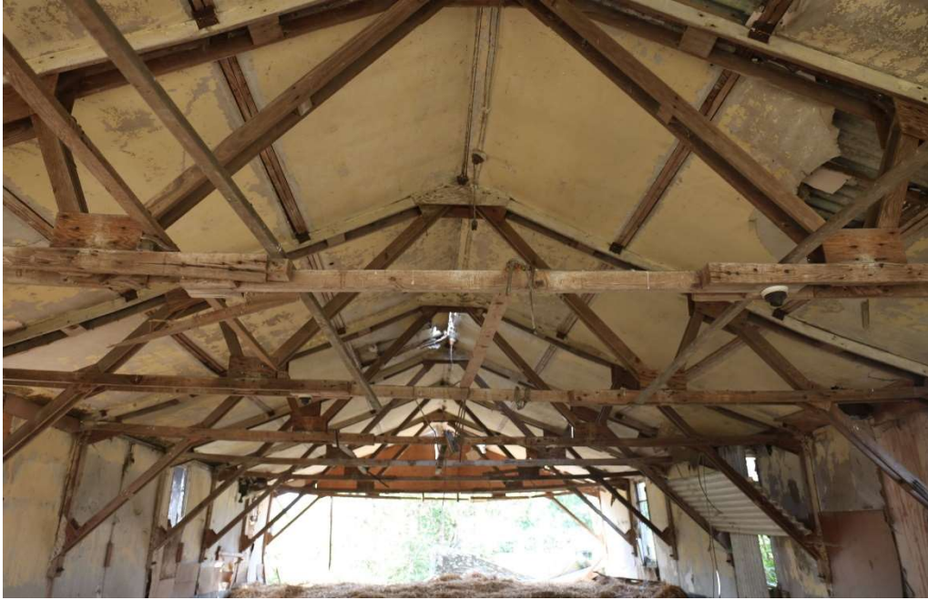
Photograph 4 Roof construction of MoWP hall hut (building 7). Photograph taken facing west.
