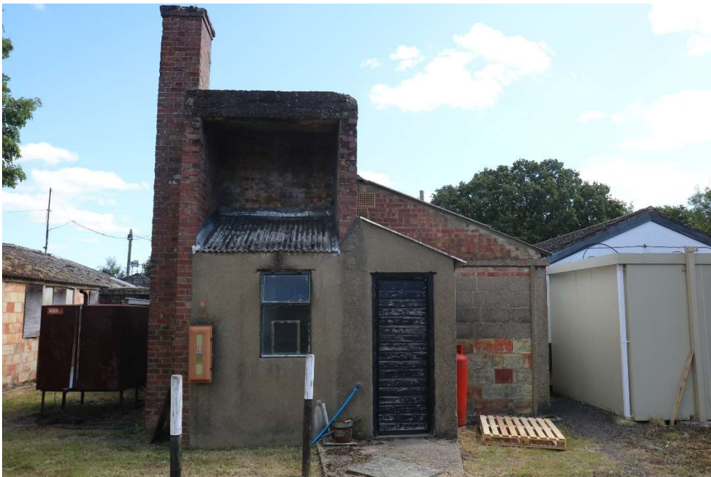
Photograph 7 Western elevation of building 2. Photograph taken facing east.
