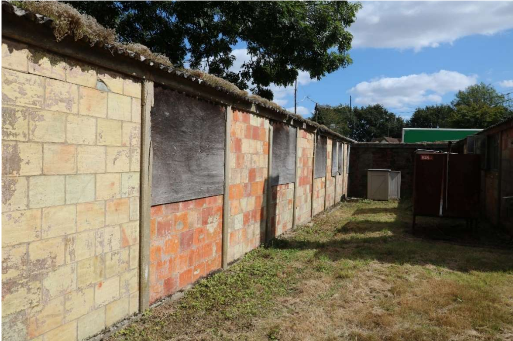
Photograph 8 Southern elevation of building 3. Photograph taken facing north-east.
