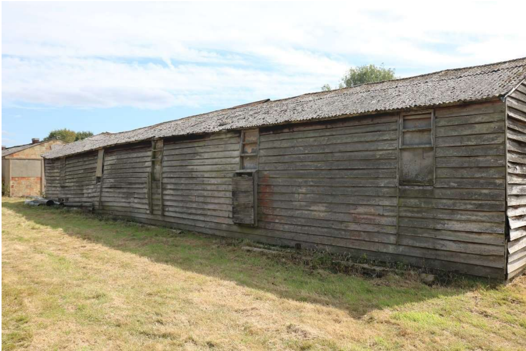
Photograph 34 Northern elevation of building 17. Photograph taken facing south-east.
