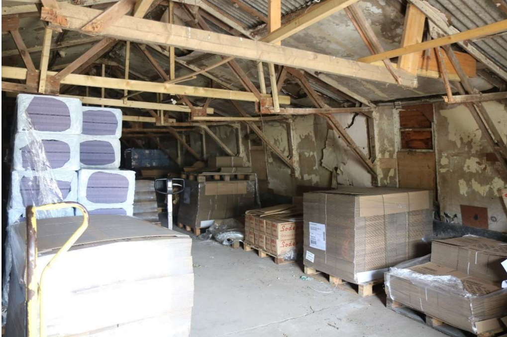
Photograph 26 Interior of building 12. Photograph taken facing north-west.
