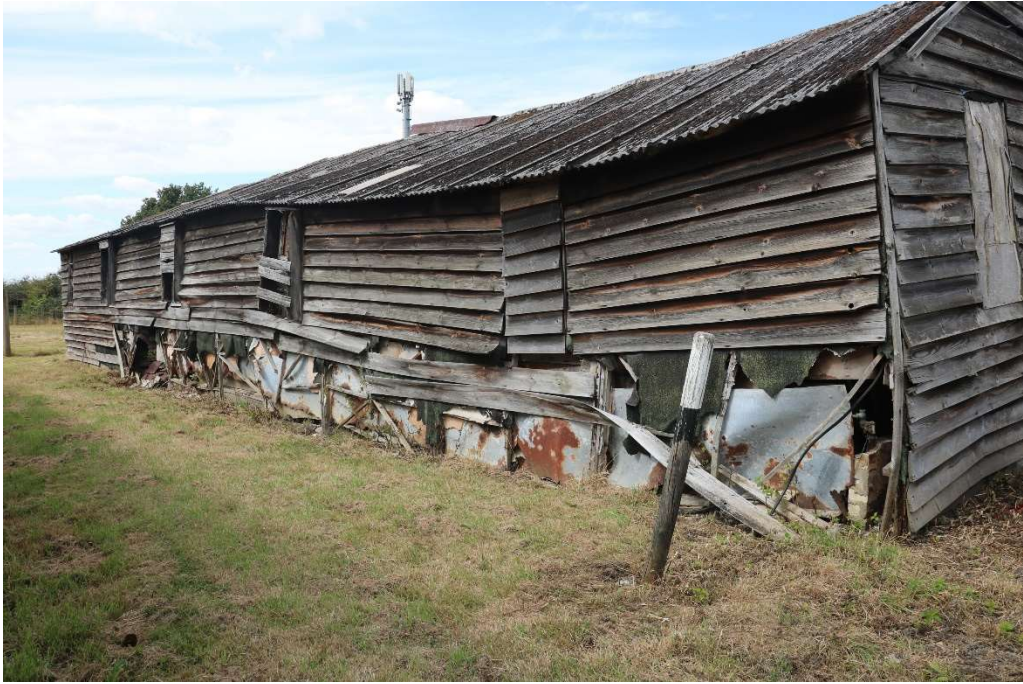
Photograph 32 Southern elevation of building 16. Photograph taken facing north-west.
