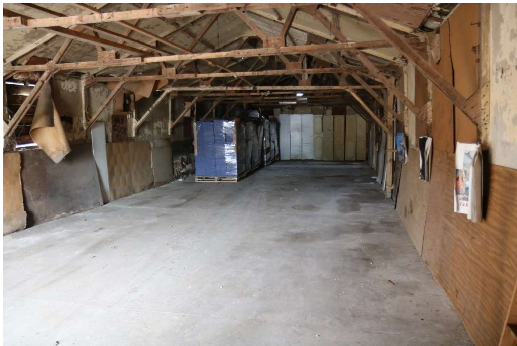
Photograph 31 Interior of building 15. Photograph taken facing south-west.
