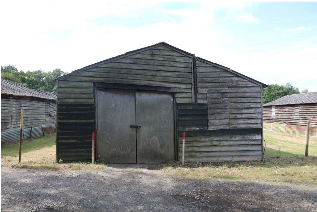
Photograph 28 Eastern elevation of building 14. Photograph taken facing west.
