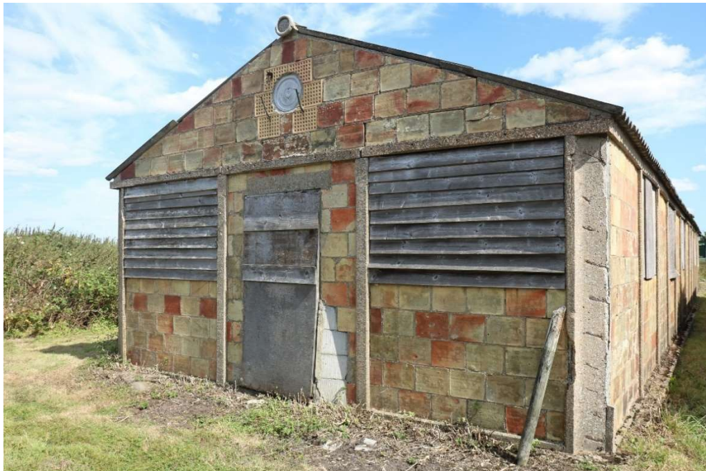
Photograph 1 Example of a MoWP standard hut (building 11). Photograph taken facing north-east.
