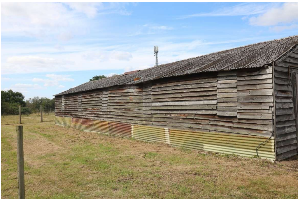
Photograph 30 Southern elevation of building 15. Photograph taken facing north-west.
