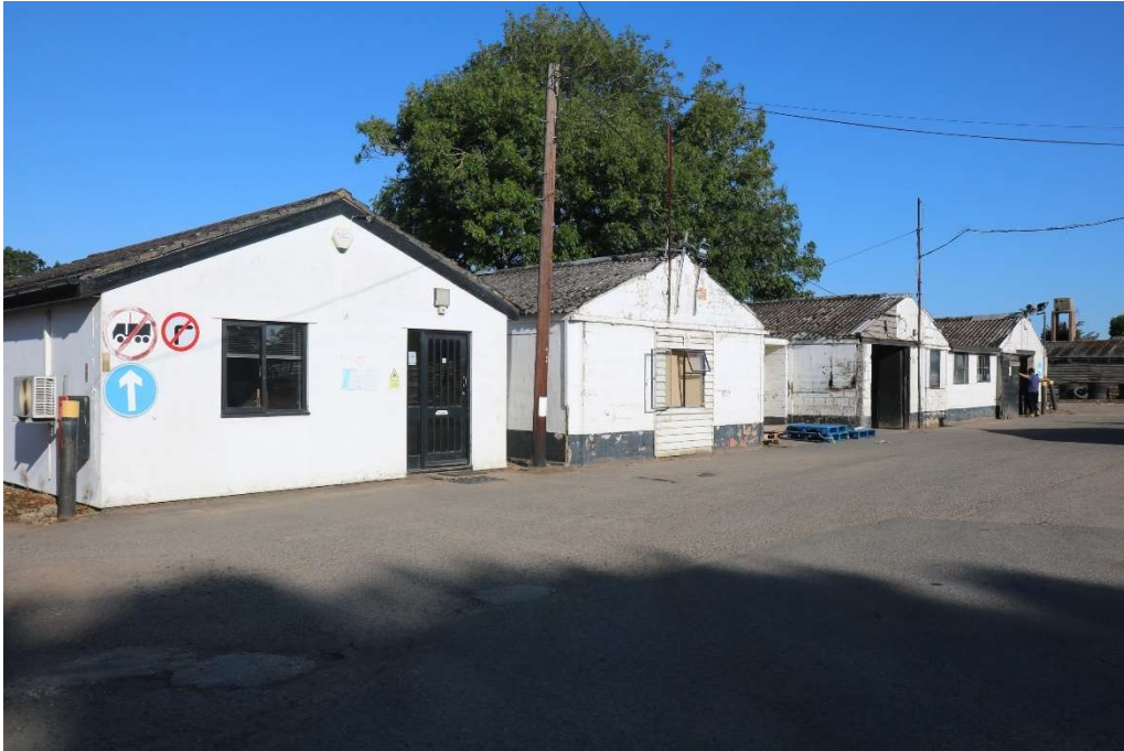
Photograph 6 Eastern elevation of building 1, 2, 3 and 4. Photograph taken facing north-west.
