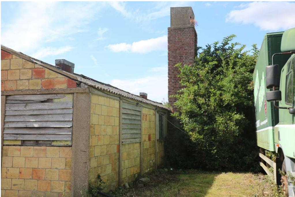
Photograph 22 Northern elevation of building 10. Photograph taken facing south-west.
