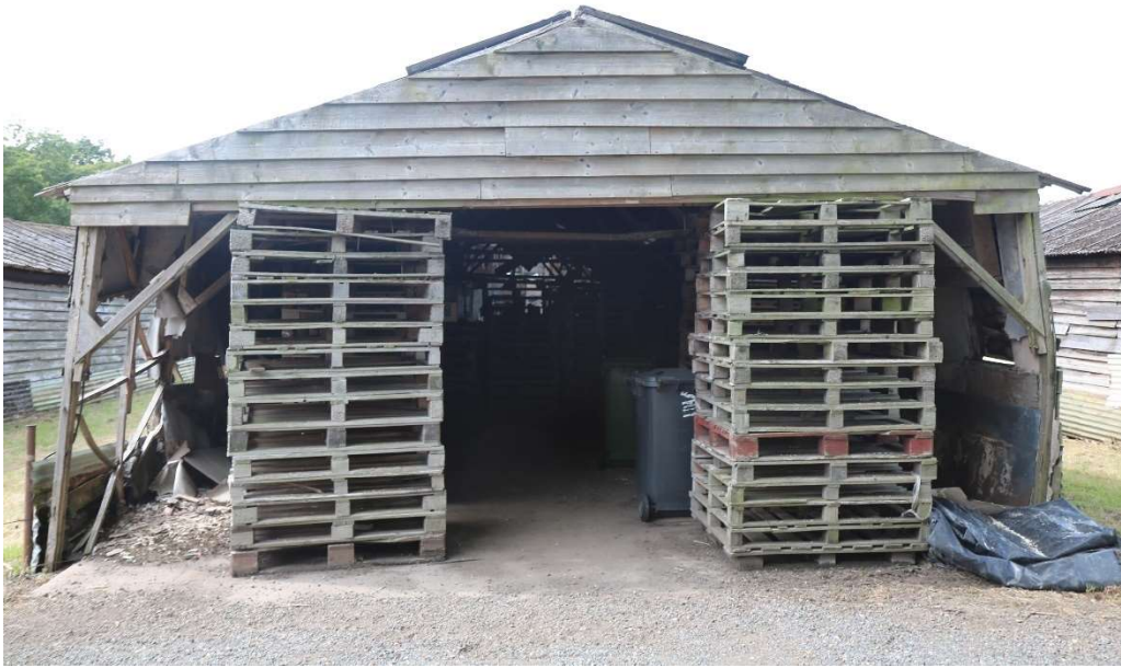
Photograph 27 Eastern elevation of building 13. Photograph taken facing west.
