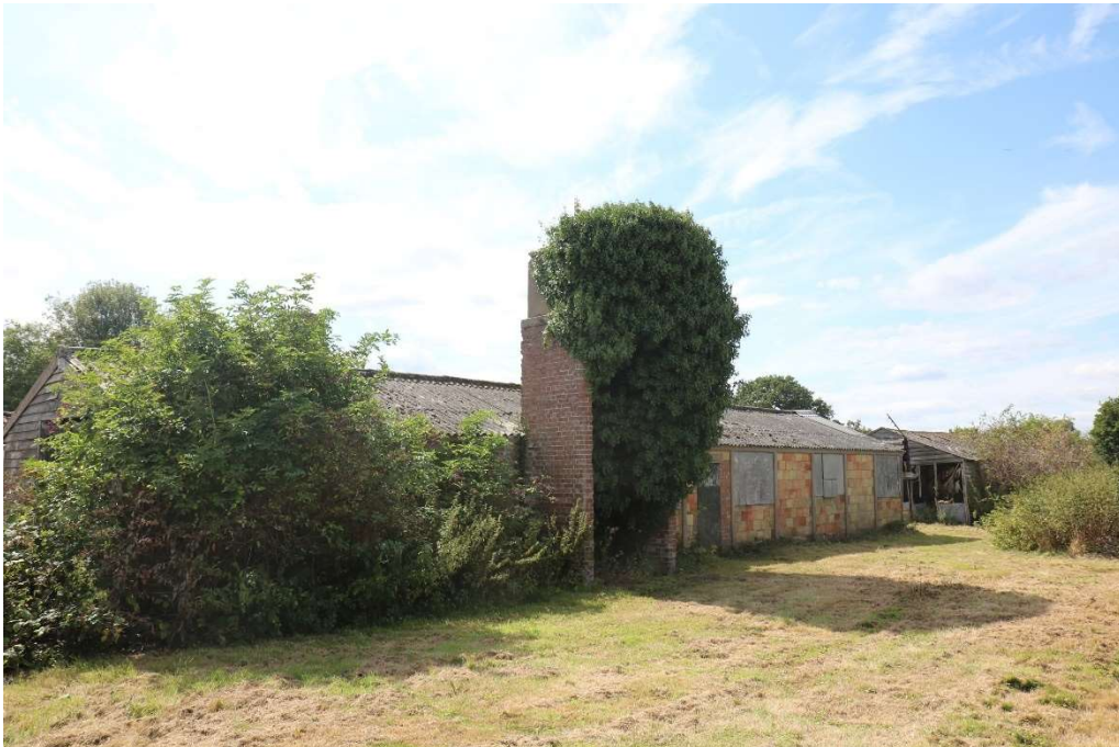
Photograph 23 Northern elevation of building 11. Photograph taken facing south-west.
