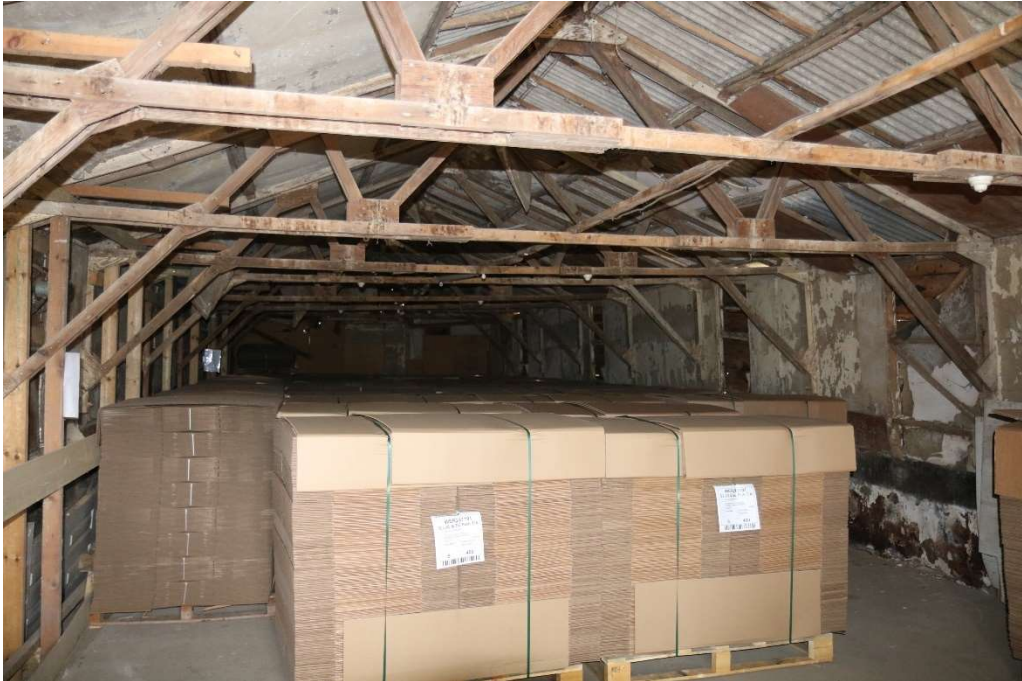
Photograph 29 Interior of building 14. Photograph taken facing north-west.
