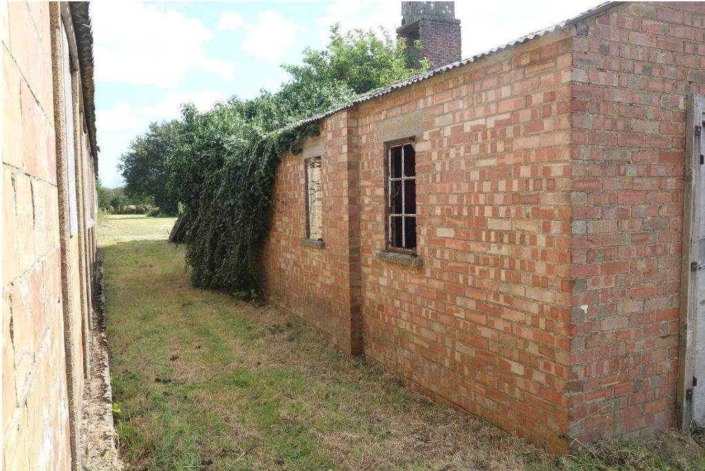
Photograph 16 Northern elevation of building 6. Photograph taken facing south-east.
