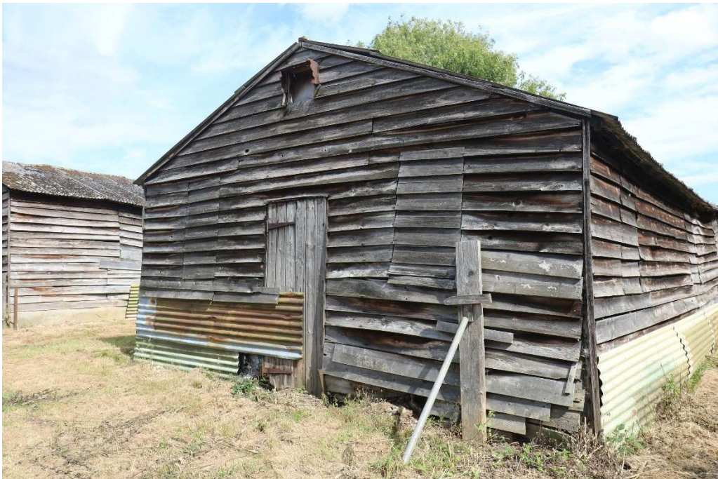
Photograph 25 Western elevation of building 12. Photograph taken facing north-east.
