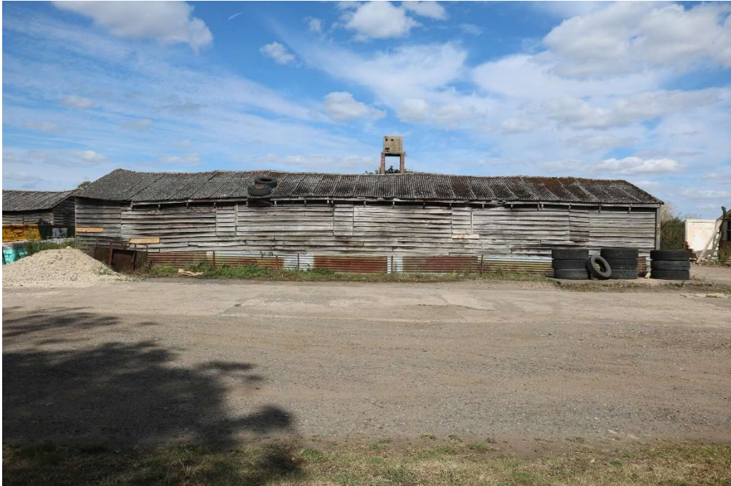
Photograph 21 Southern elevation of building 9. Photograph taken facing north.
