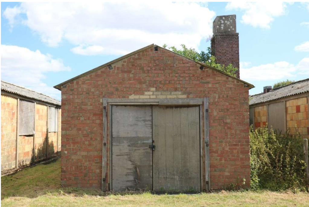
Photograph 15 Western elevation of building 6. Photograph taken facing east.
