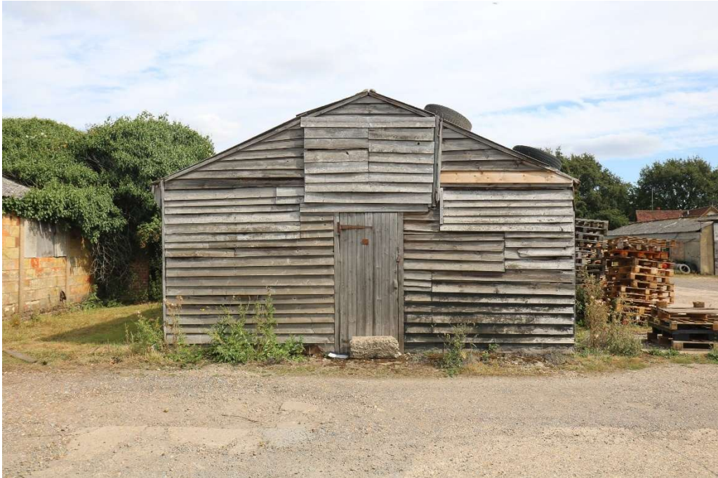
Photograph 37 Western elevation of building 19. Photograph taken facing east.
