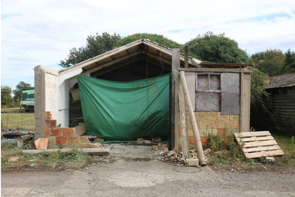
Photograph 36 Western elevation of building 18. Photograph taken facing east.
