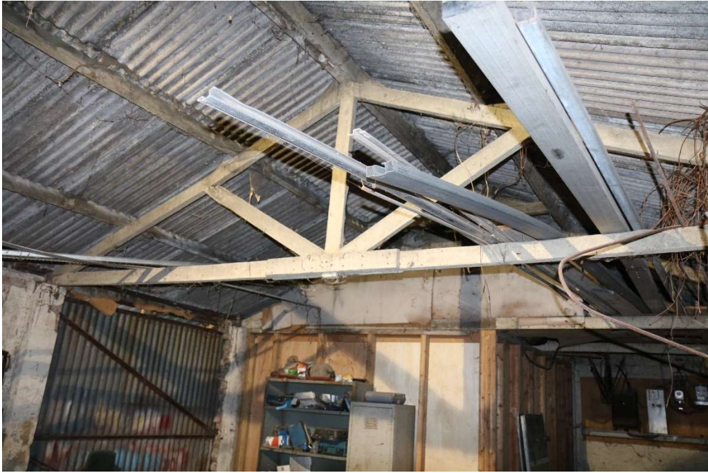
Photograph 14 Roof construction of rear extension of building 5. Photograph taken facing north-east.
