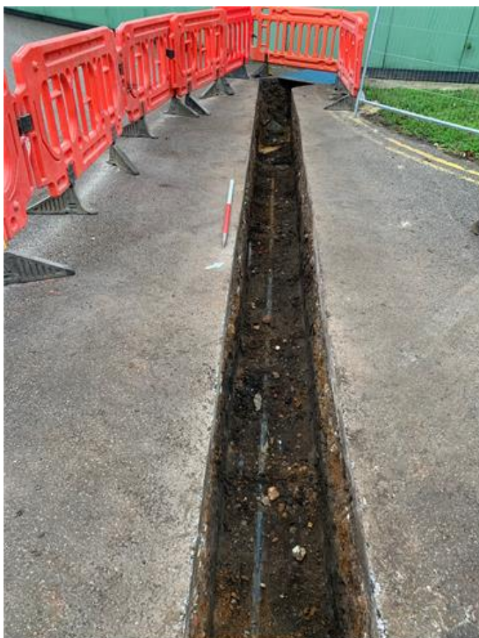
Photograph 4 Trench and old gas pipe, facing north-west.
