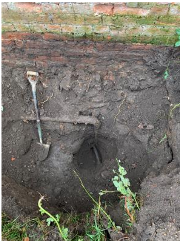
Photograph 1 Gas pipe near East Hill House wall, facing north.
