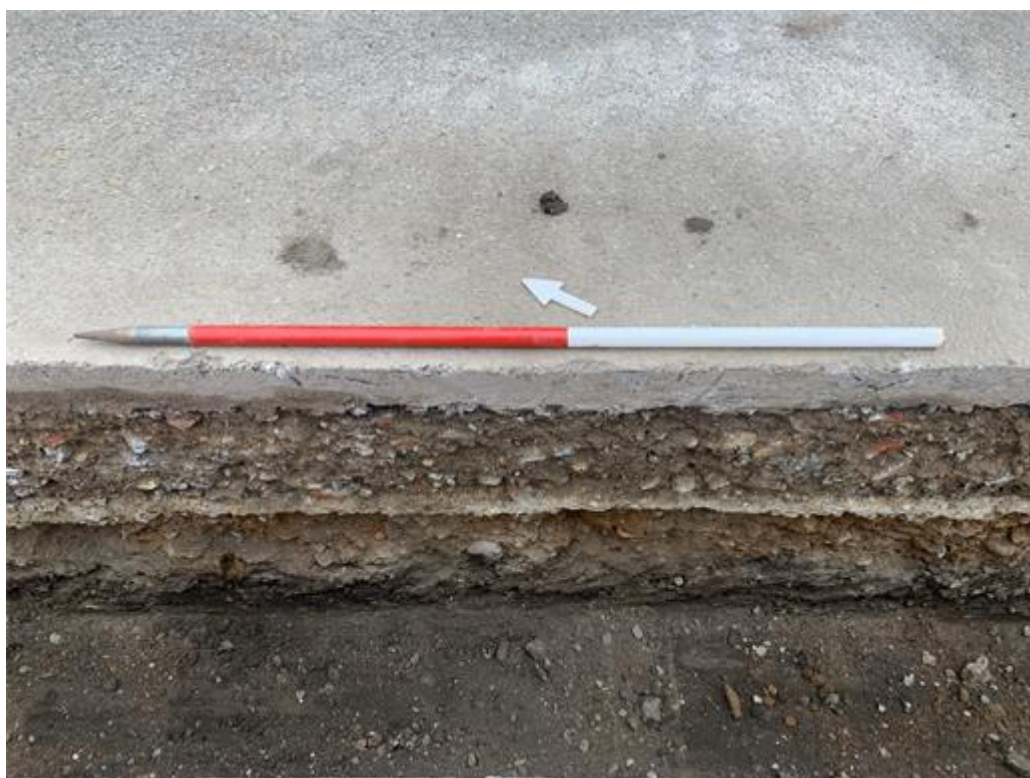
Photograph 5 Representative-section 2 facing north-east.
