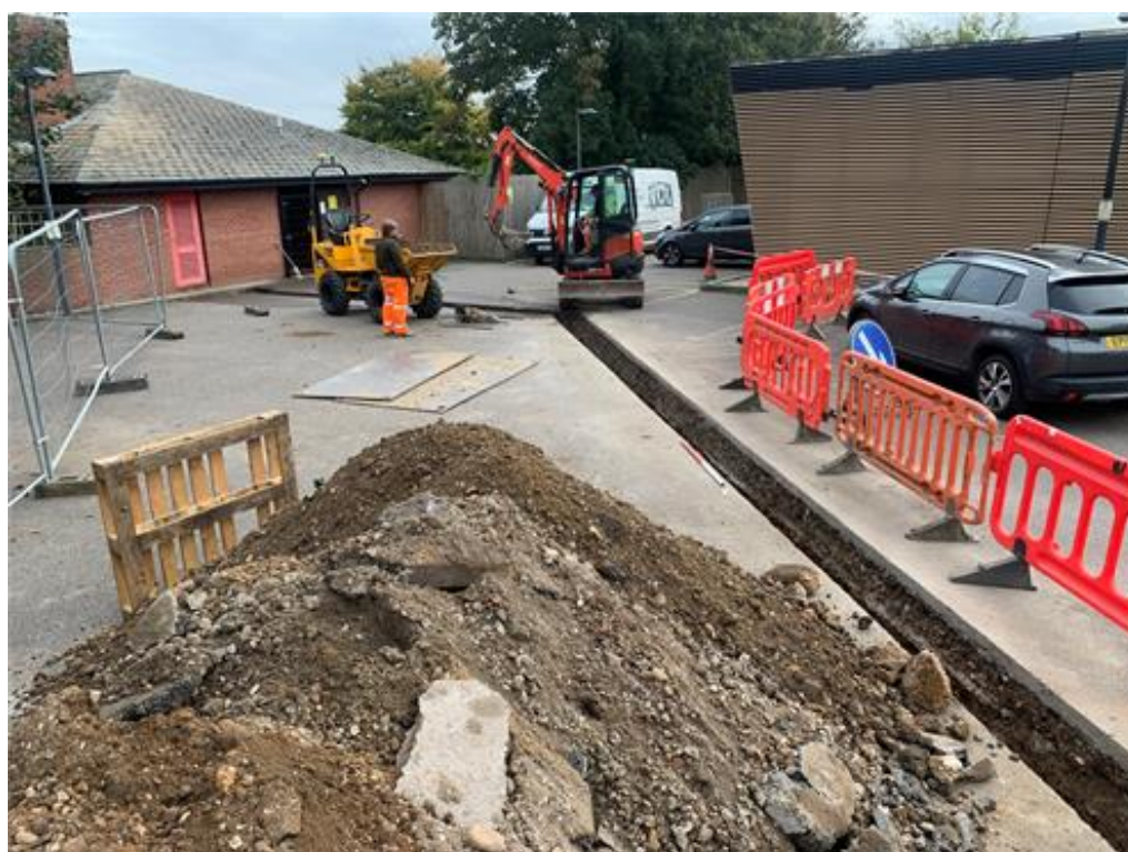
Photograph 6 Overall view of site, looking south-east.
