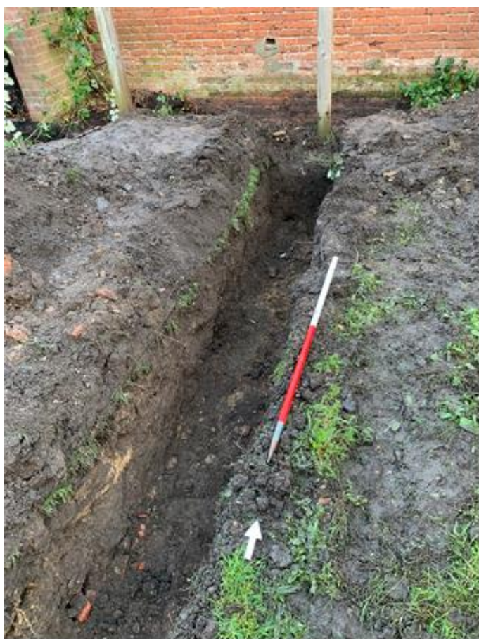
Photograph 2 Pipe trench, facing north.
