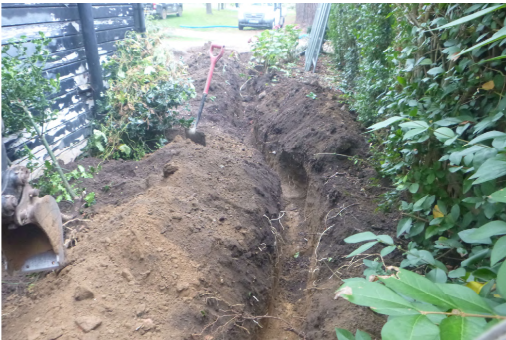
Photograph 2 The trench to the rear of the toilet block, view east.
