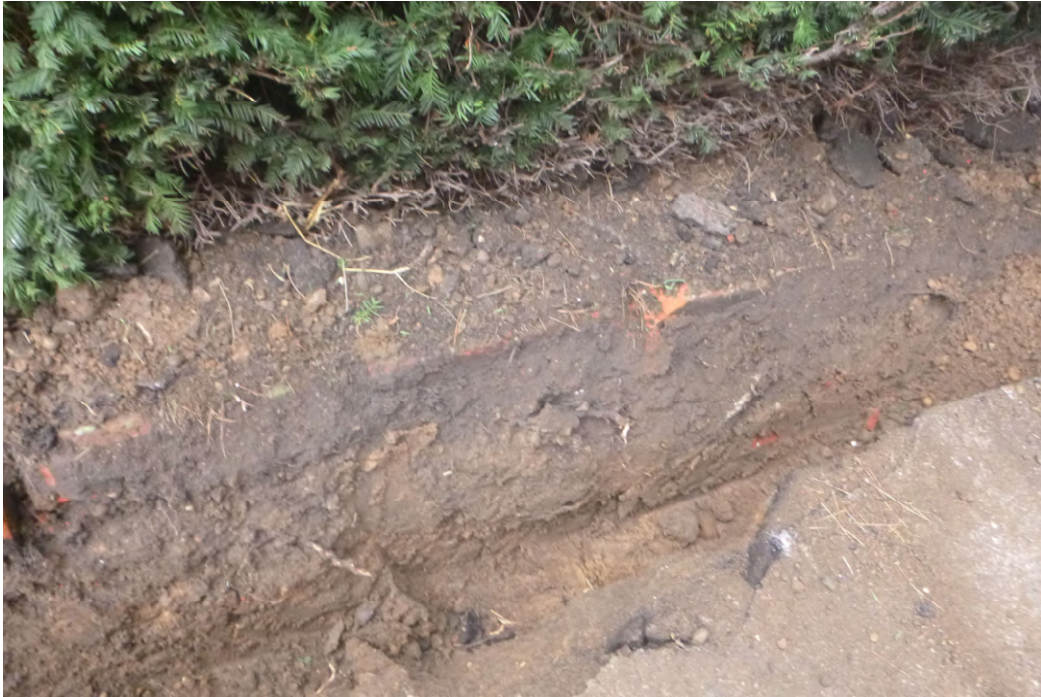
Photograph 1 The trench along the footpath, view west.
