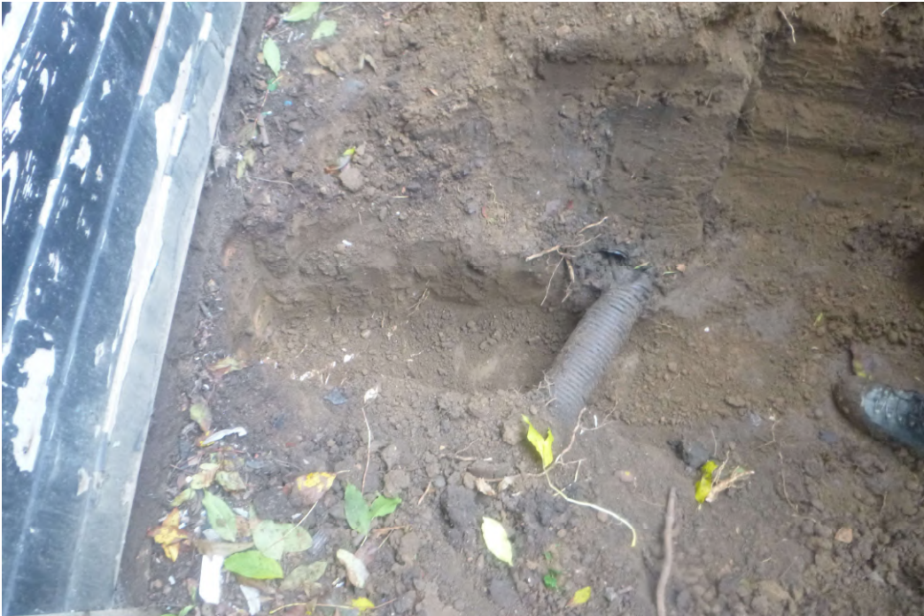
Photograph 4 The trench to the rear of the toilet block, view east.
