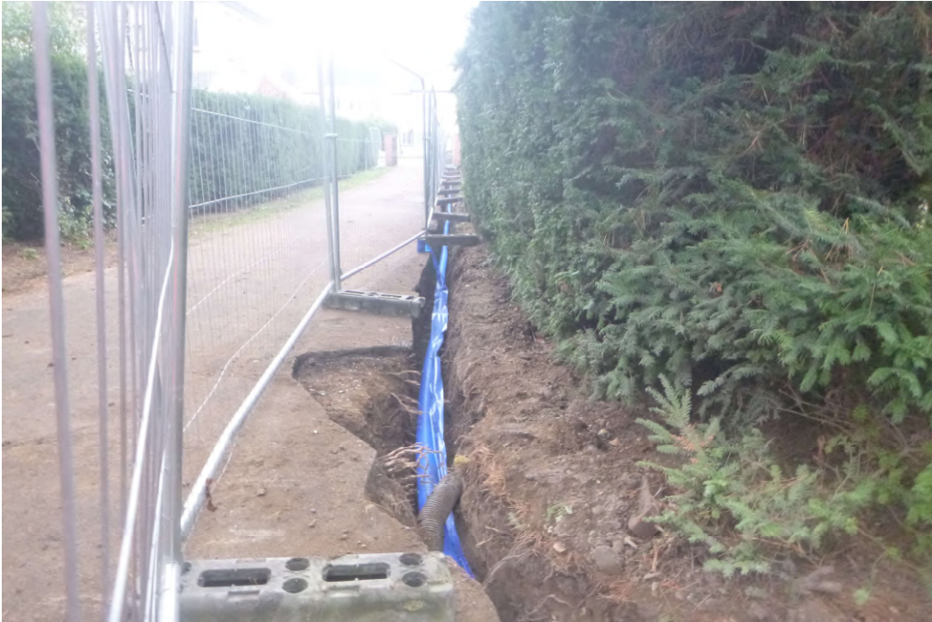
Photograph 3 The trench along the footpath with replacement pipe laid, view south.
