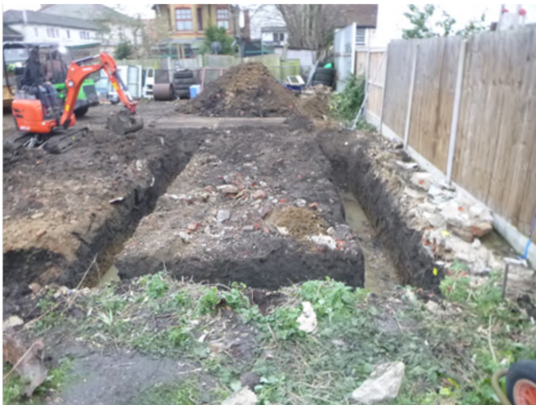
Photograph 2 Foundation trenches, looking east.
