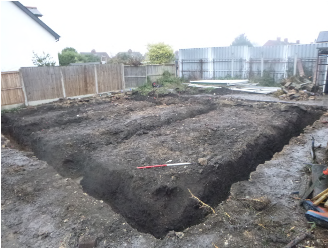
Photograph 4 Foundation trenches, looking north-west.
