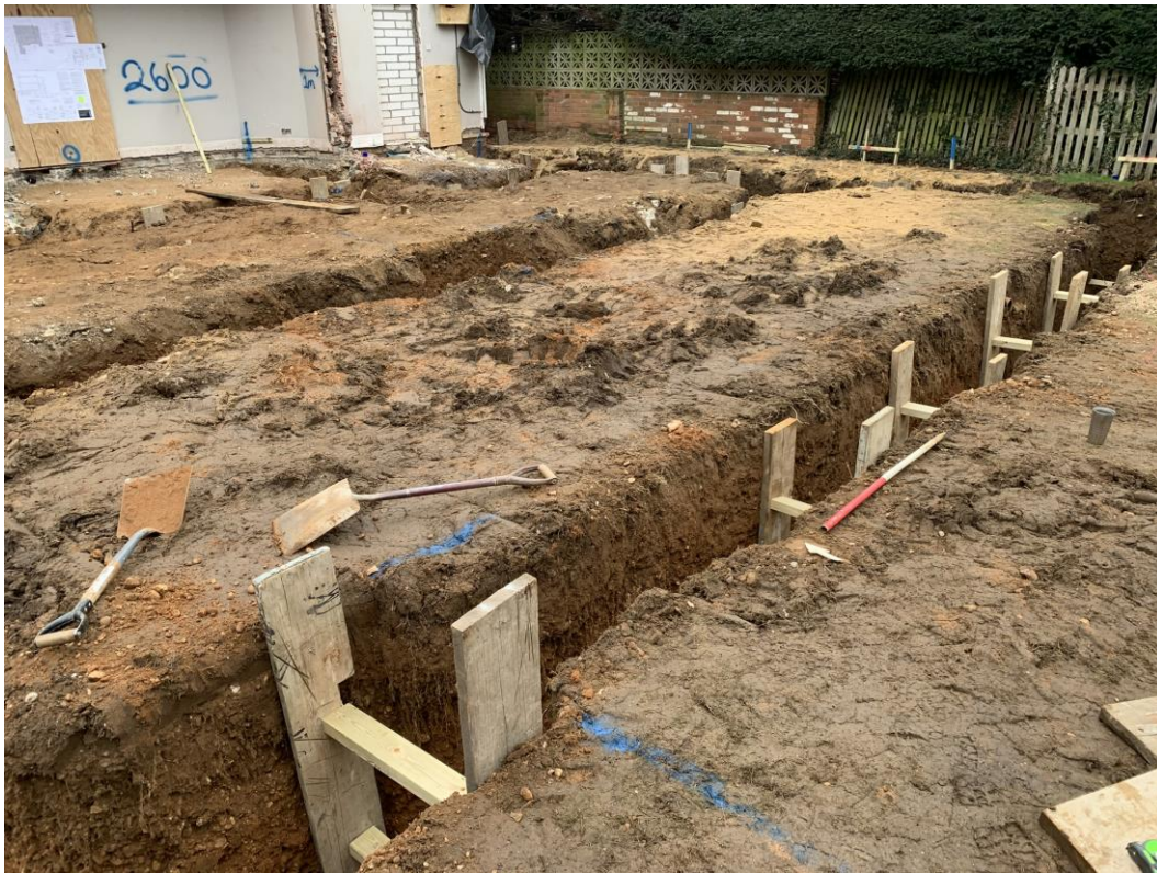
Photograph 3 Foundation trenches and shuttering in place, looking north-east.
