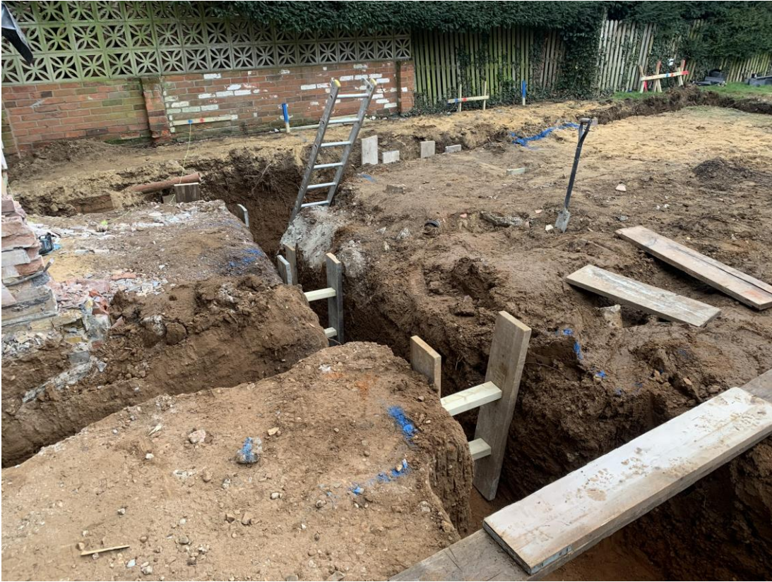
Photograph 1 Foundation trenches and shuttering in place, looking east.
