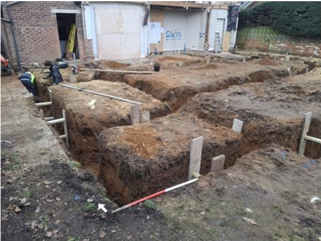
Photograph 2 Foundation trenches, looking north-east.
