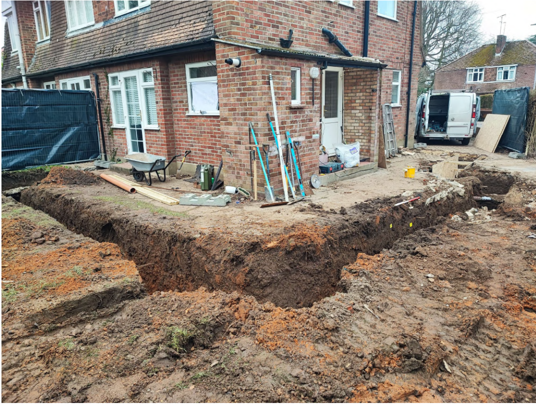
Photograph 2 The foundation trench, looking north-north-west.
