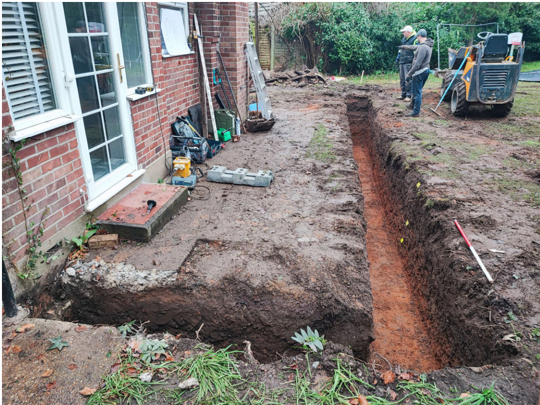
Photograph 1 The southern half of the foundation trench, looking west-south-west.
