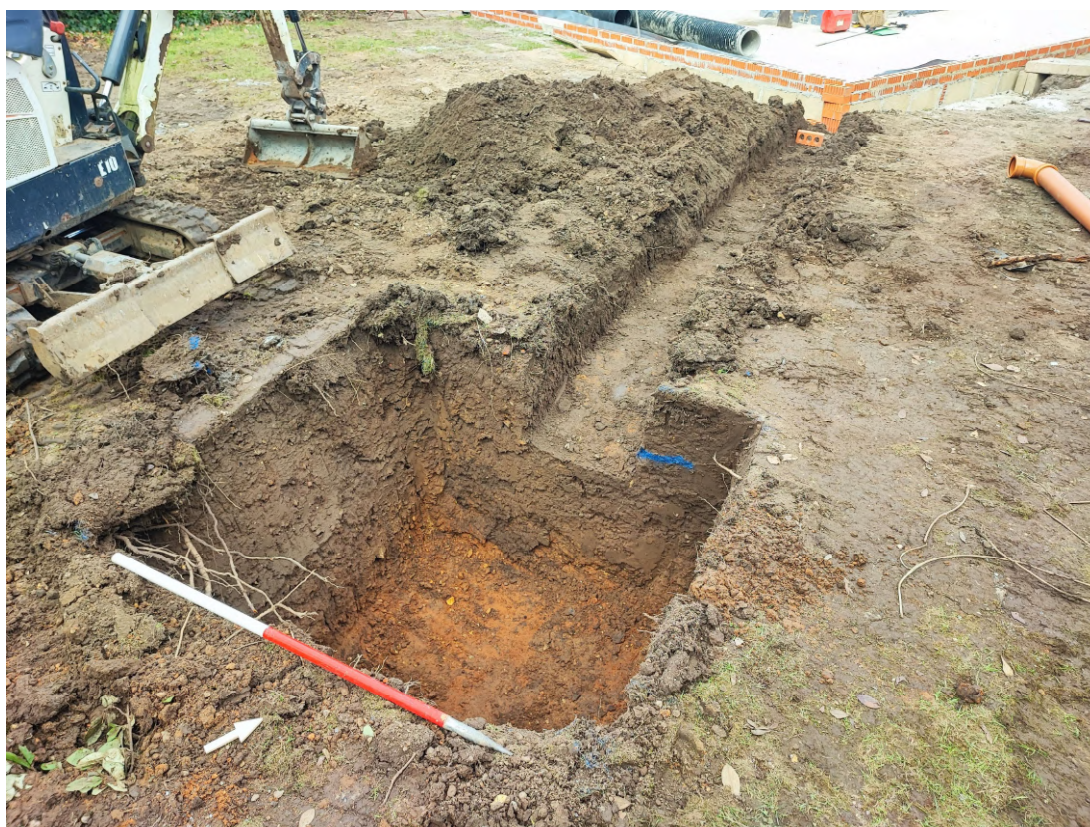
Photograph 6 The soakaway and drainage trench, looking north-west.
