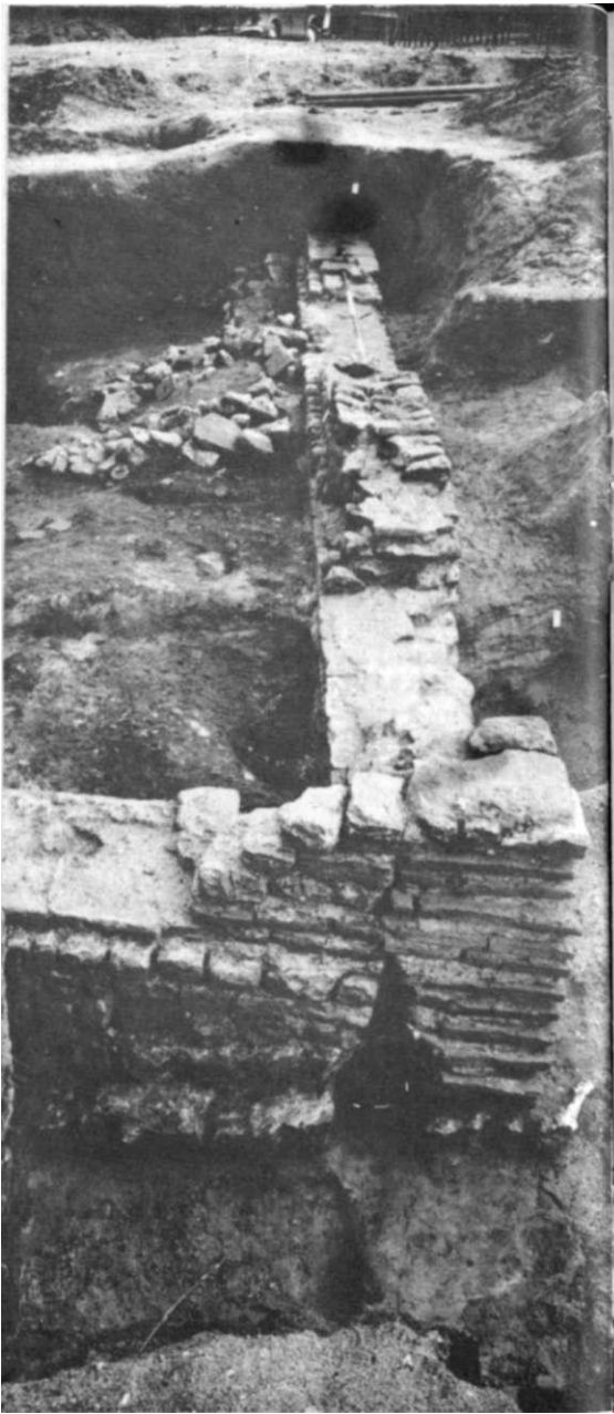
View of the south-west corner of the church during excavations in 1977. The walls are built of Kentish ragstone and layers of Roman tile. When the Police Headquarters are built on this site it is hoped that the re-excavated church will be preserved in a permanent display there.
