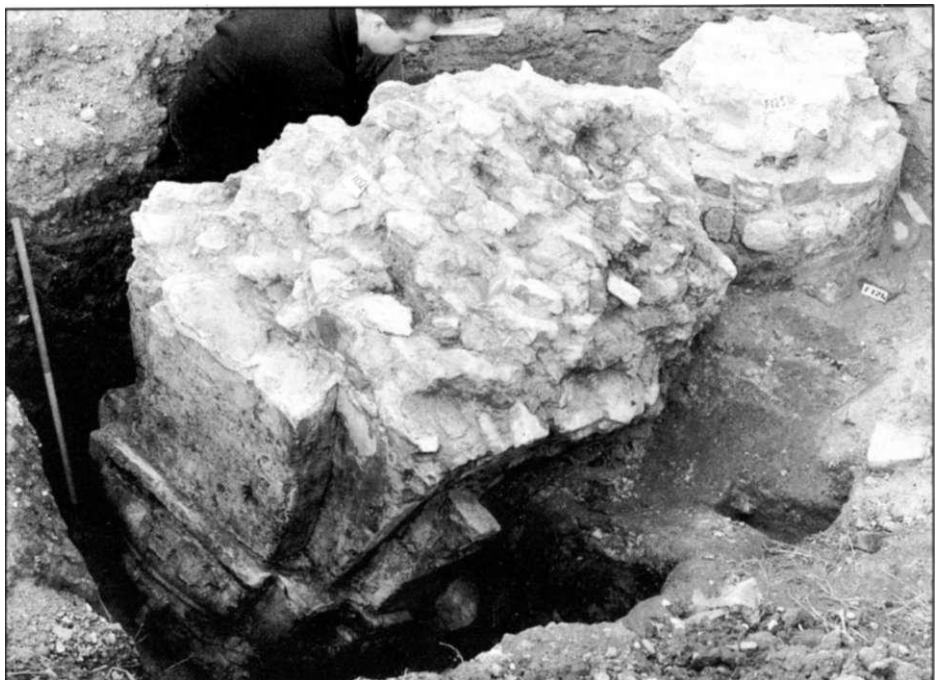
The collapsed section of column in the crypt. The stump of column on the crypt floor is visible to the rear right.
