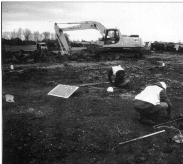
Excavations in progress at Turner Rise
