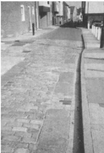
You will sometimes find old paving like this. These are hard stone blocks (usually granite) cut with a chisel into rectangles or wedges. These 'setts', as they are called, can be anything from 15 to 45 centimetres deep.
